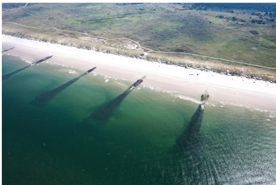
Figure 5.1 Groyne at Vlieland, in front of beach with vegetated dunes.
