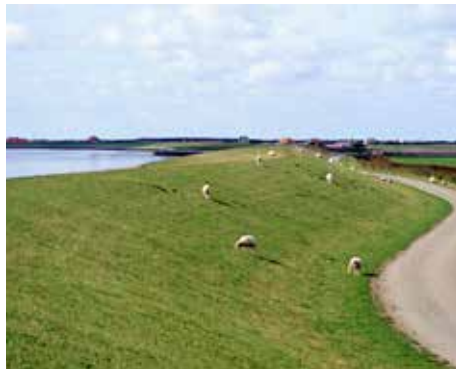
Figure 19: Dike combined with agriculture
