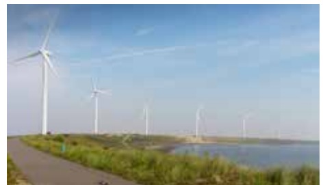
Figure 16: Wind turbines on the dike
