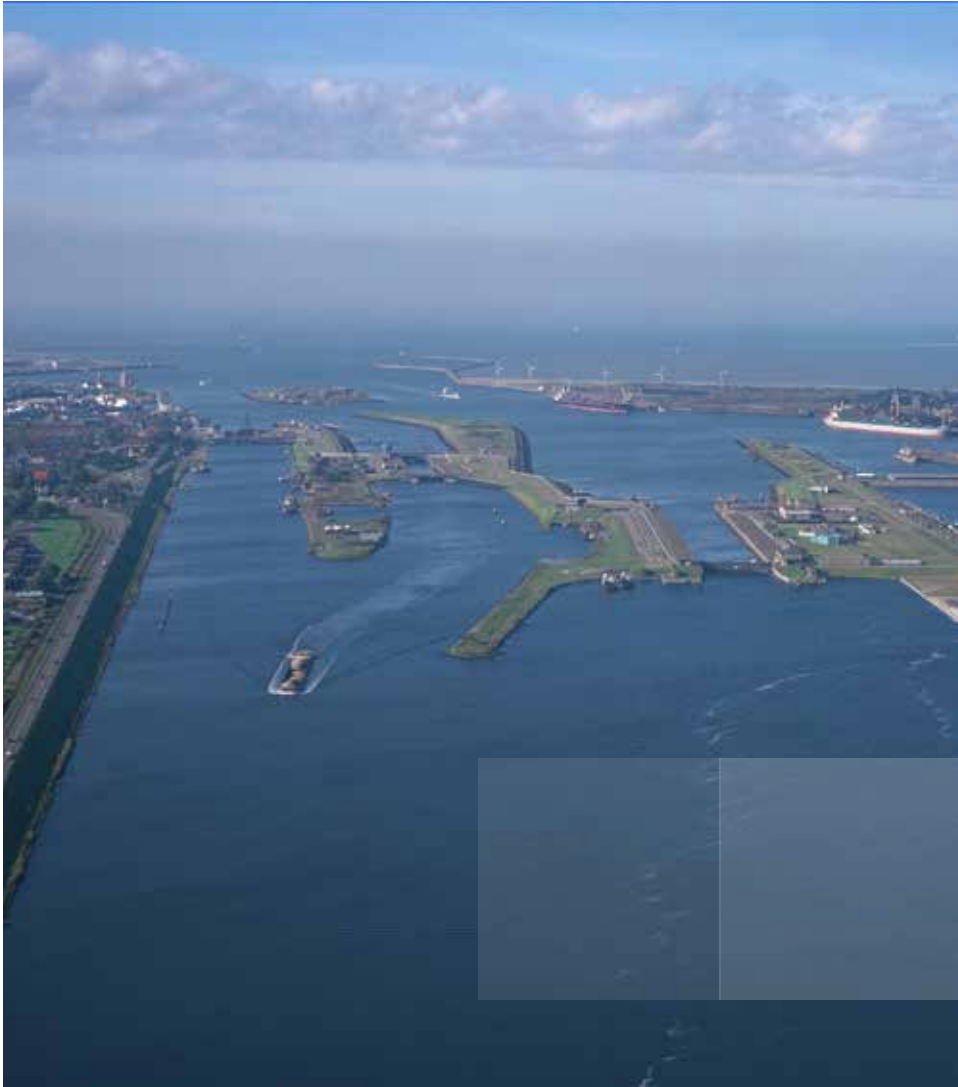
Figure 29: The locks at IJmuiden
