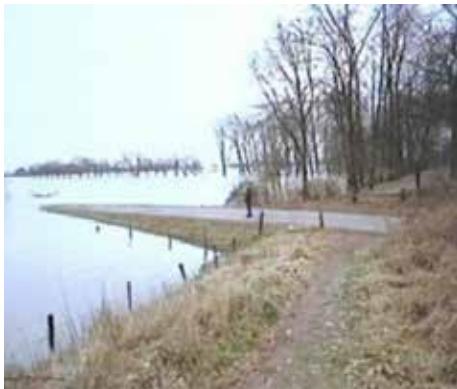
Figure 20: The tree dike in Wilp forms an ecological corridor
