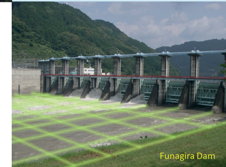
Downstream of Funagira Dam. The green lines show an example of coarse grid shape.
