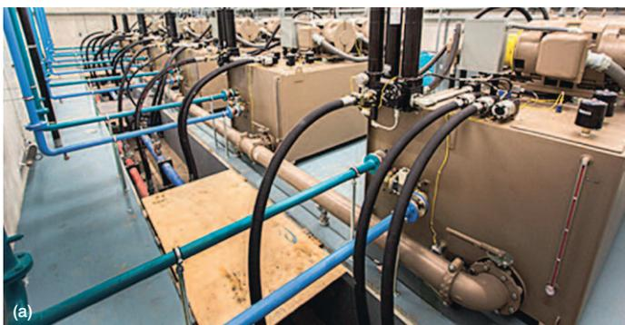
(a) hydraulic power units for wave generator
