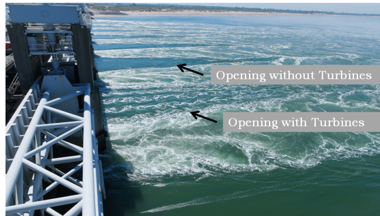
Figure 2.13: Photograph taken from above Roompot 8. Eastern Scheldt barrier and turbine wake interaction during ebb, photograph taken by M. Verbeek (2017)
