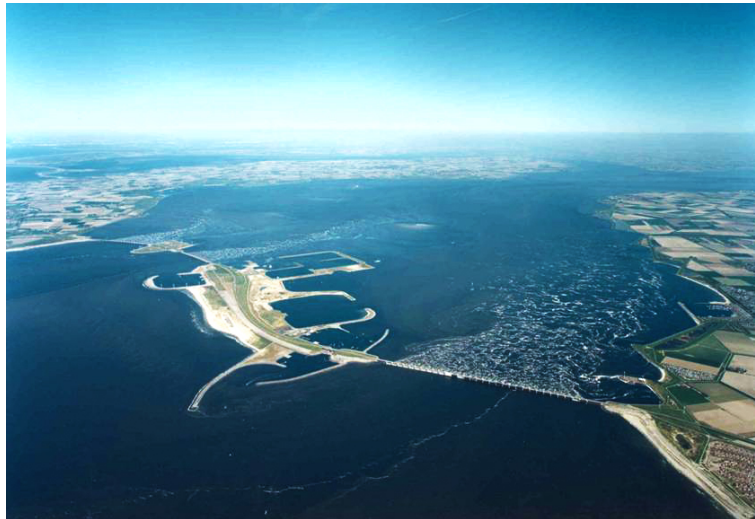
Figure 2.12: Aerial photograph of flow through the Eastern Scheldt barrier during flood (Biesboer, 2011)
