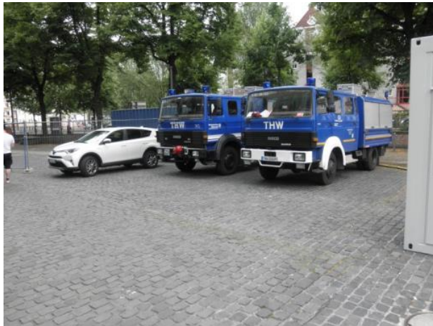
THW is contracted for the flood wall construction in Rheinauhafen
