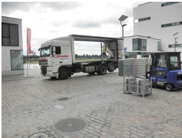
Supply of the flood wall elements with hired trucks etc.
