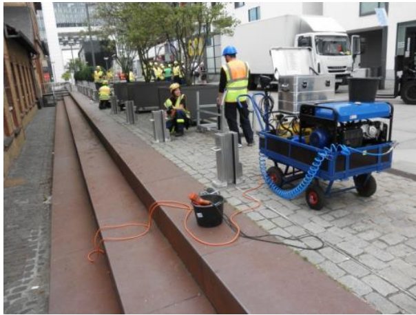
Fixing the poles
