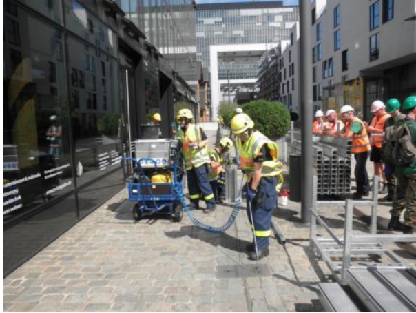
Cleaning the bolt holes with air pressure
