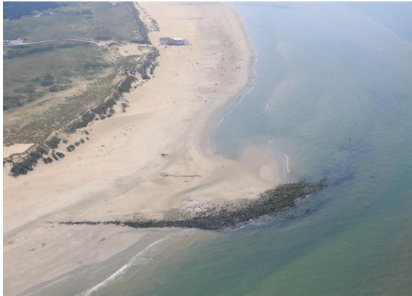
Figure 2.18. Break water near JarKus transect 3000240 at Ameland West. The break water clearly extends more seaward than the adjacent areas.
