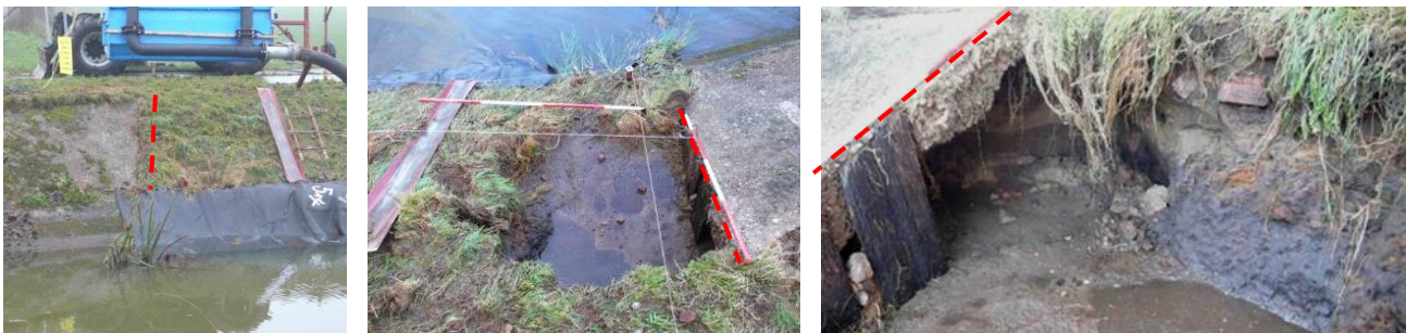
Figure 16. Impression of Test Section Ol.2. Left: initial condition. Middle and right: condition after 500 impacts.
