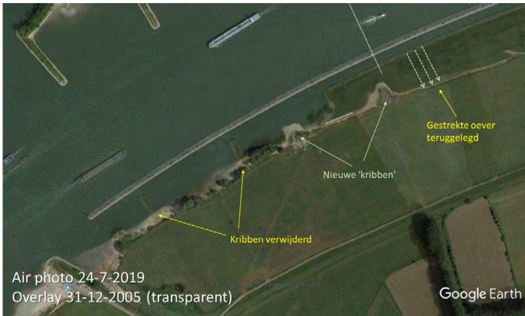
Figure 23 Google Earth® aerial photograph of auxiliary channel at Wamel at RKM 912.5. Aerial photograph of 2019 and 2005 are overlaid to see the former location of the bank line that was set backward, and the location of the new groynes relative to the old groynes. The lower left corner is the ferry crossing Tiel-Wamel.
