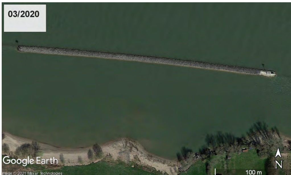
Figure 67 Satellite image of the upstream end of the longitudinal training wall at Wamel in 2020.
