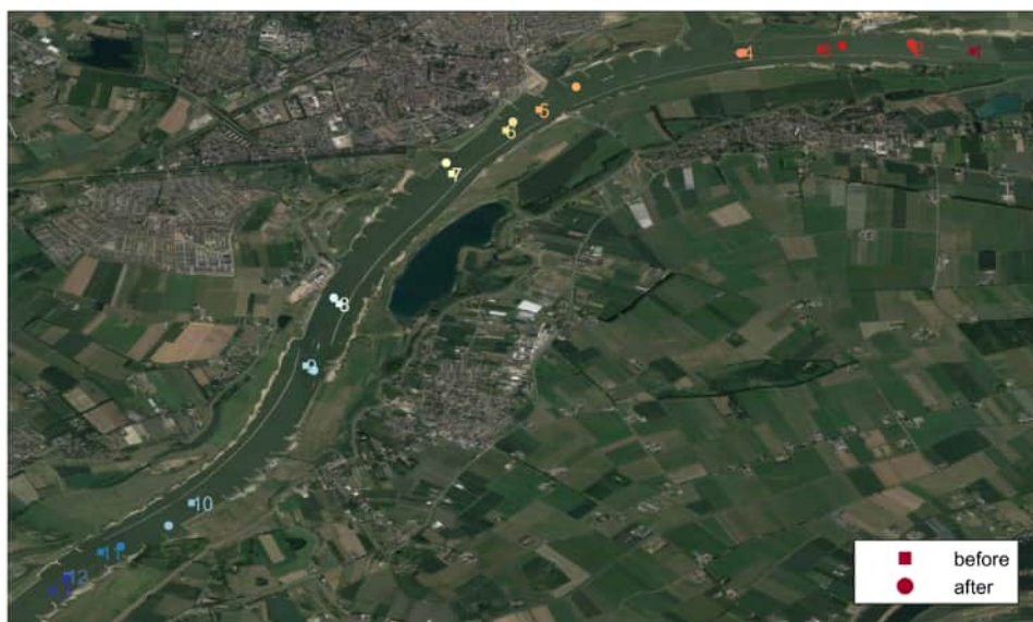
Figure 3.7 Location of the cross-sectional measurements before and after intervention for condition 4. . For each measurement before construction (square marker with number) the matched measurement after construction (circle marker) is given the same color.
