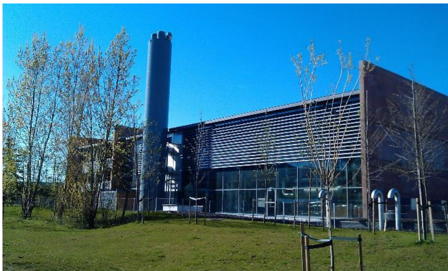
Figuur 15: Referentie centrale warmtepomp: Drammen Fjernvarme AS (bron: STAR Renewable Energy)
