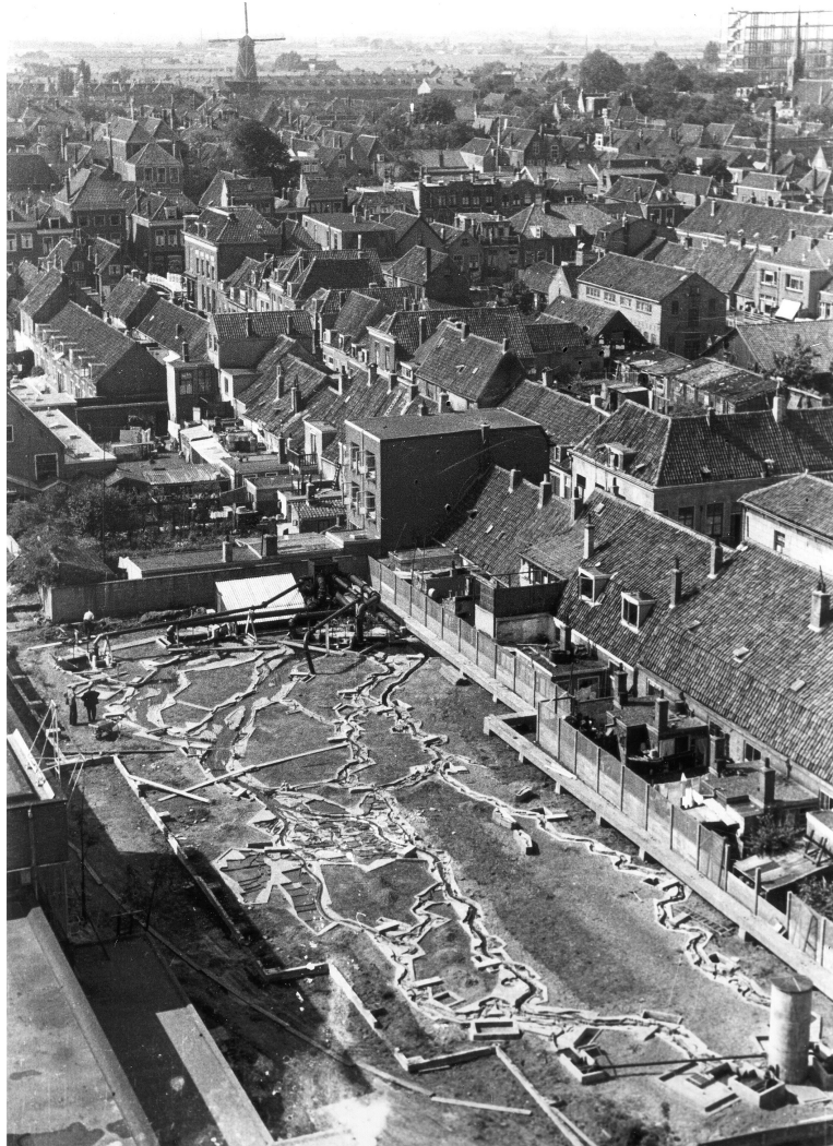
Figure 1 Picture of the scale model of the Dutch Rhine-Meuse branches built by the Waterloopkundig Laboratorium in the centre of Delft in 1950. The model was built in the Schuttersveld and the picture was taken from Het Raam. The church on the top right corner is the Lutherse Kerk (also known as Saint George's Chapel) and the windmill on the top left is Molen de Roos. Flow goes from bottom to top. The right-hand branch is the Lek. The second branch starting to count from the right is the Waal. The third one is the Meuse. The upstream boundary is approximately at Wijk bij Duurstede and Tiel. The Biesbosch is visible in the centre of the domain on the left.
