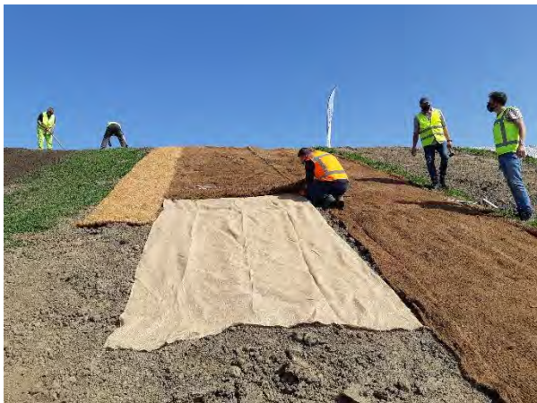
Figure 2.13 Placing of a jute mat with wooden pins
