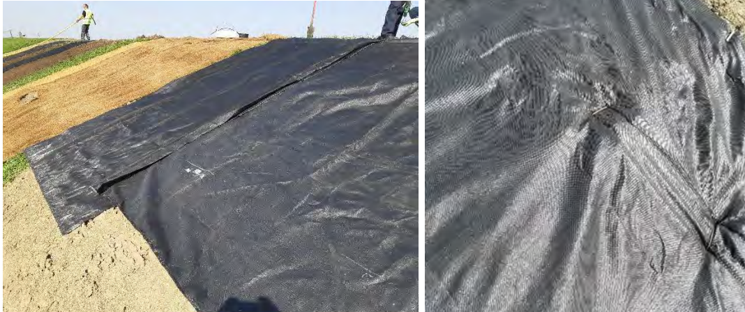
Figure 2.14 The recently sown clay top-layer is covered by PE180 geotextile, using U-pins and small T-pins.
