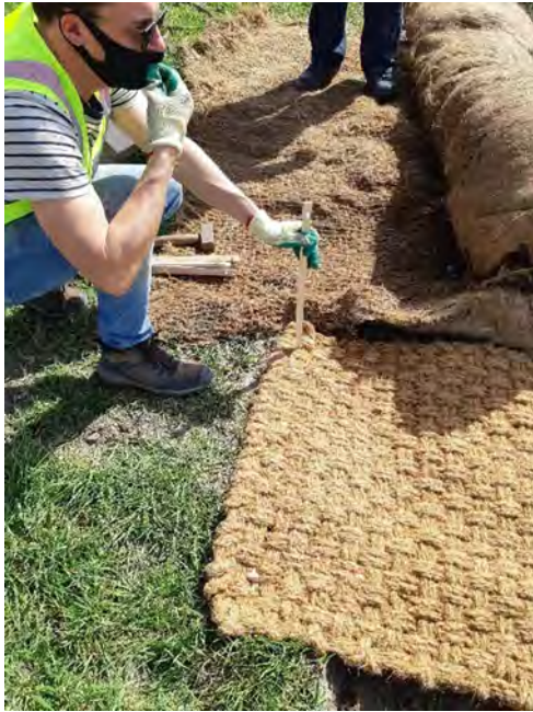
Figure 2.12 Fixing the coco mats with wooden pins
