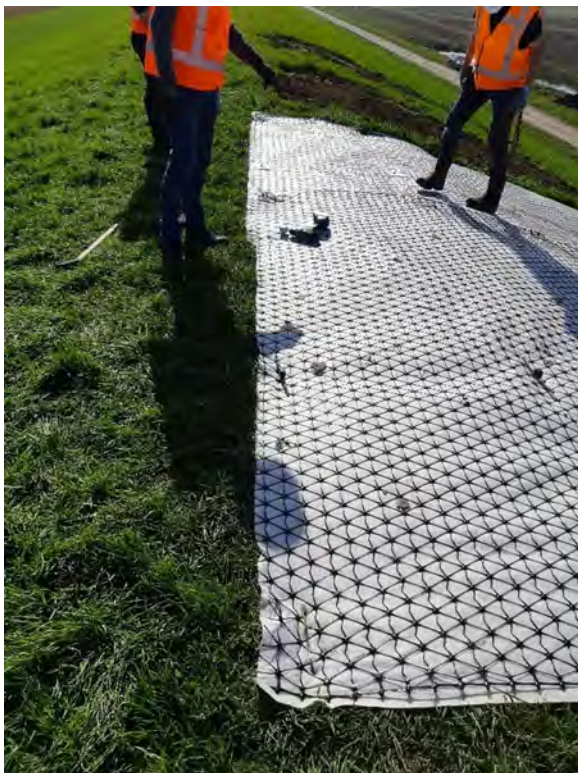
Figure 2.6 View on the different fixation pins of the panel
