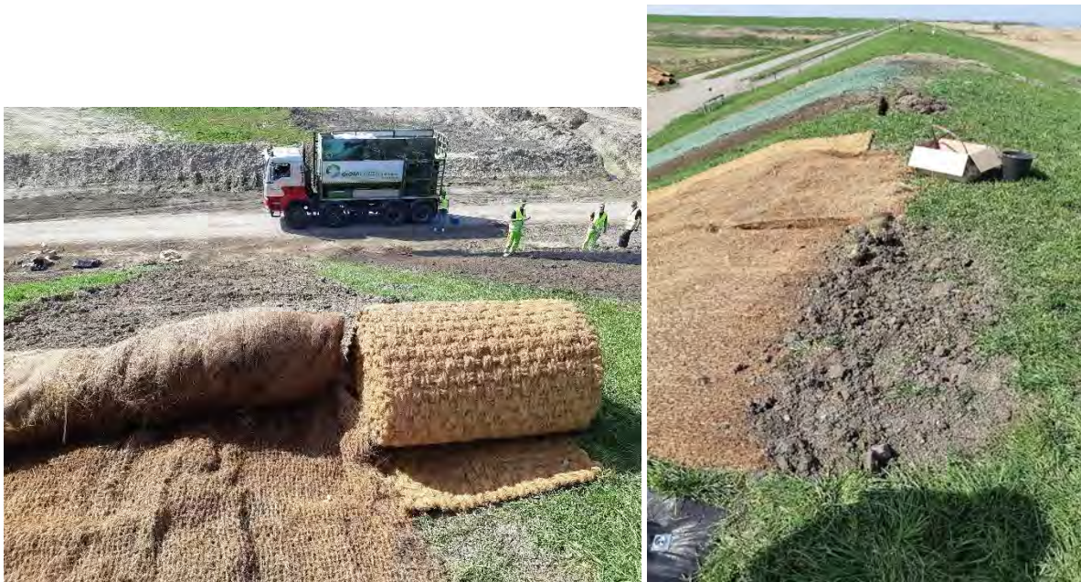
Figure 2.11 Two different coco mats are placed without an overlap
