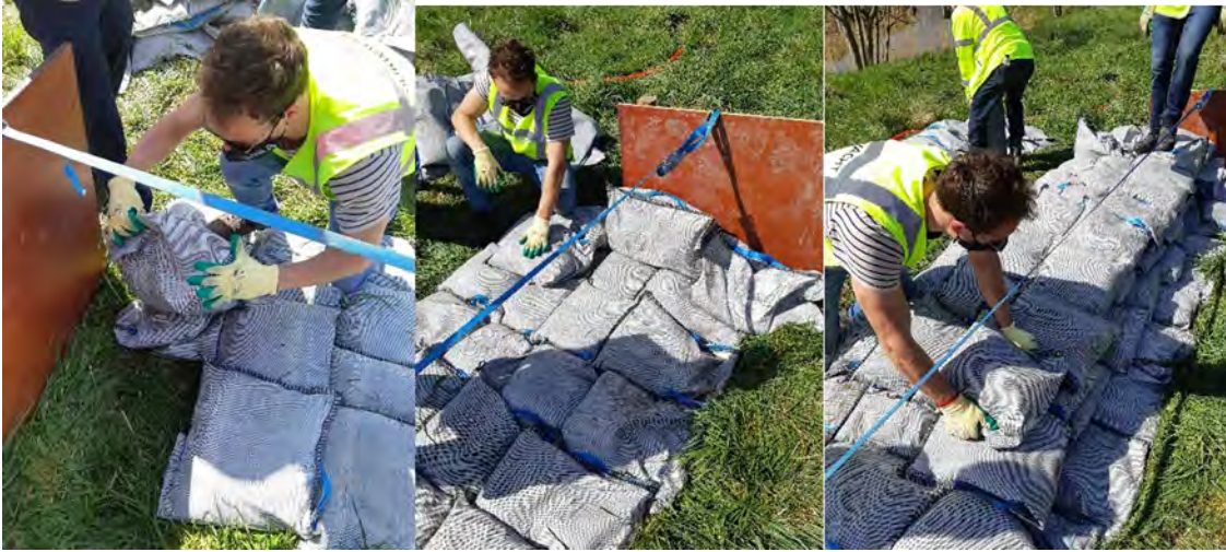
Figure 1.4 Building up a sandbag dam with PP-bags
