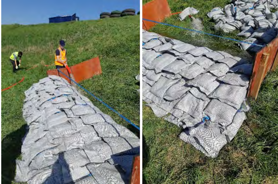
Figure 1.3 traditional built-up dam
