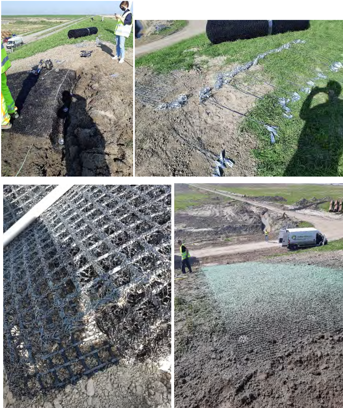
Figure 2.15 Placing of a turf mat with Grippe Terra-Lock anchors and pins.
