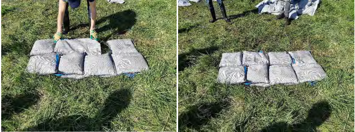
Figure 1.10 Correct placement of the PP-sandbags
