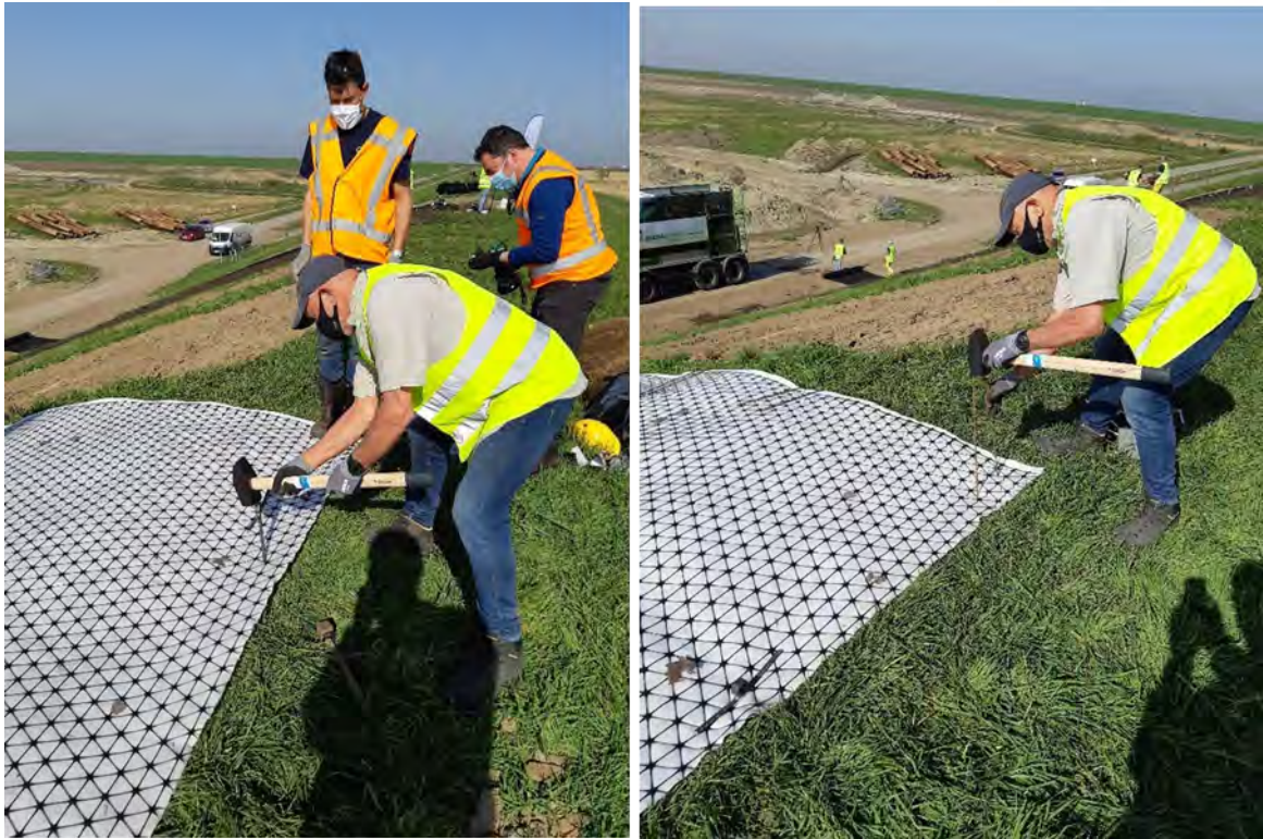
Figure 2.5 Fixing the Tensar panel with 5 rows of different types of pins (left: Y-pin, right: U-pin)
