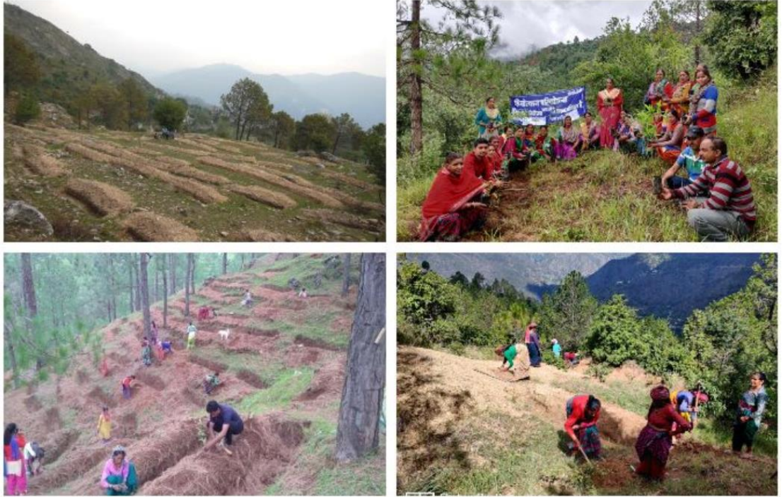
Figure 3-16 Examples of methods to improve recharge capacity in a spring watershed. The examples show different methods: To slow down the surface runoff (top row) or capture the surface runoff water in small ponds for infiltration (bottom row).
