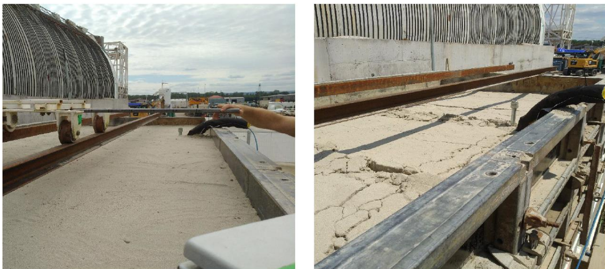
Figure 22: Settlement before (left) and after advance (right)
