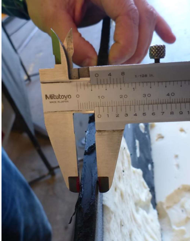
Figure 97: Wall thickness of nearly 9 mm in the stressed area
