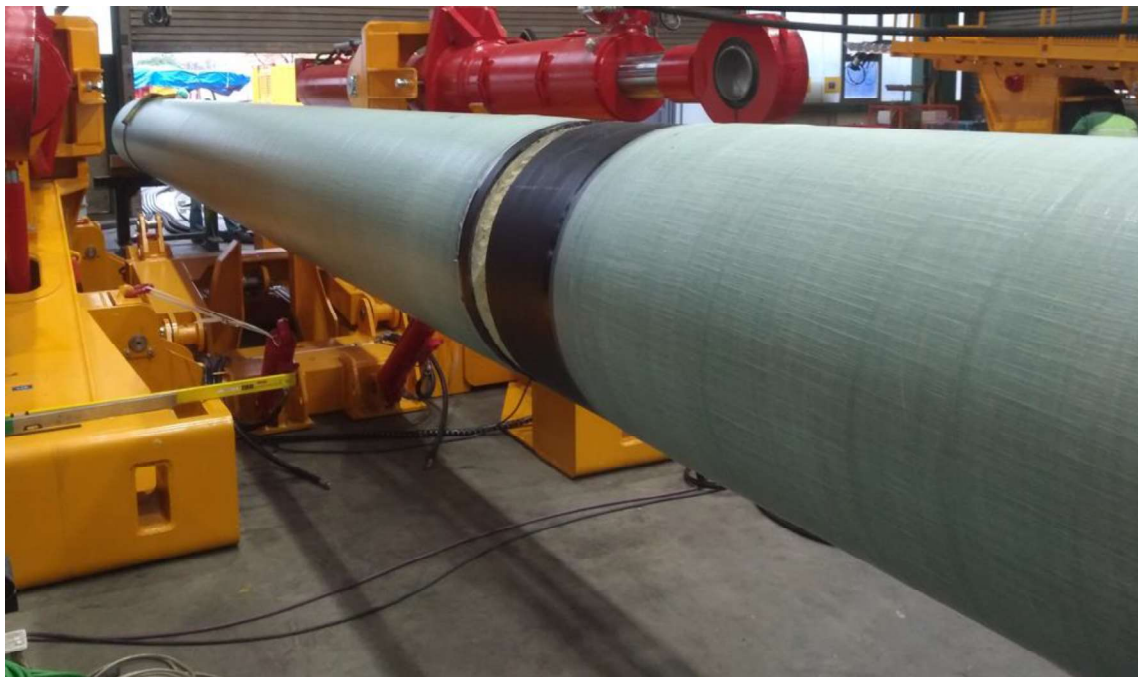
Figure 45: Installation of HDPE GRP pipe
