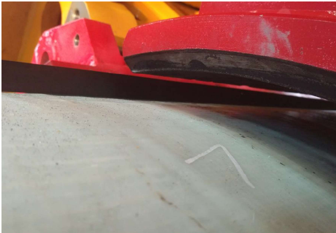
Figure 54: No damage visible after 200 bar clamping pressure
