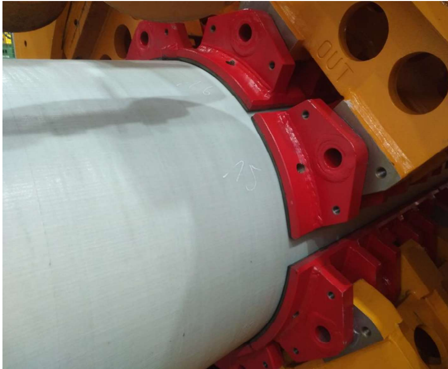
Figure 46: Clamping of HDPE GRP pipe
