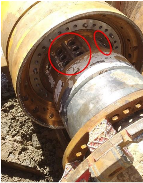
Figure 26: Grain limiter on the suction box
