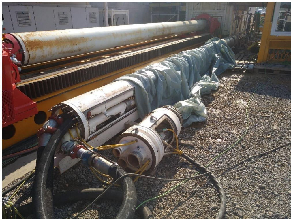
Figure 4: Pipe thruster, thrust pipe, EPP
