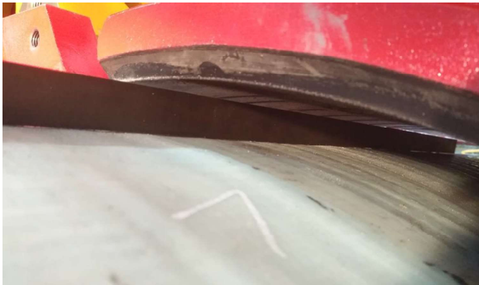
Figure 52: No damage visible after 130 bar clamping pressure
