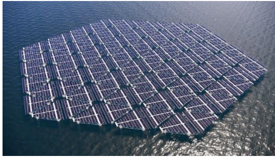
Figure 1: A comparison between the SolarDuck design (a) (10 MW – triangular elevated solution existing of 96 connected platforms, source: SolarDuck) and the OceanSun design (b) (7,8 MW – 12 floating membranes of 0,65MW per membrane. source: https://oceansun.no/our-products/ ). The SolarDuck OFPV are elevated above the sea level, while the OceanSun OFPV are floating on the water surface.
