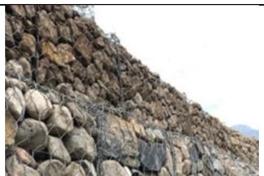
Figure 6: Example – Gabion wall
