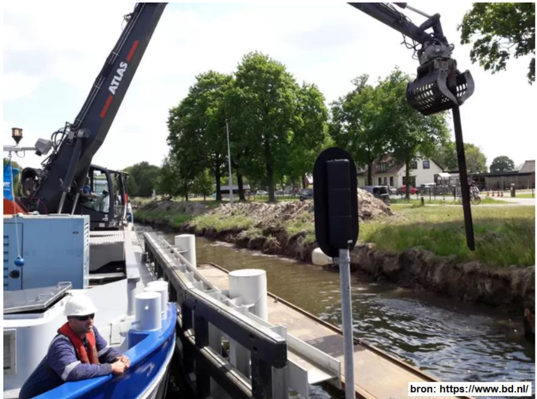
Figure 2 Replacement of sheet piles along the Wilhelminakanaal. Extraction of a sheet pile (May 26, 2020).
