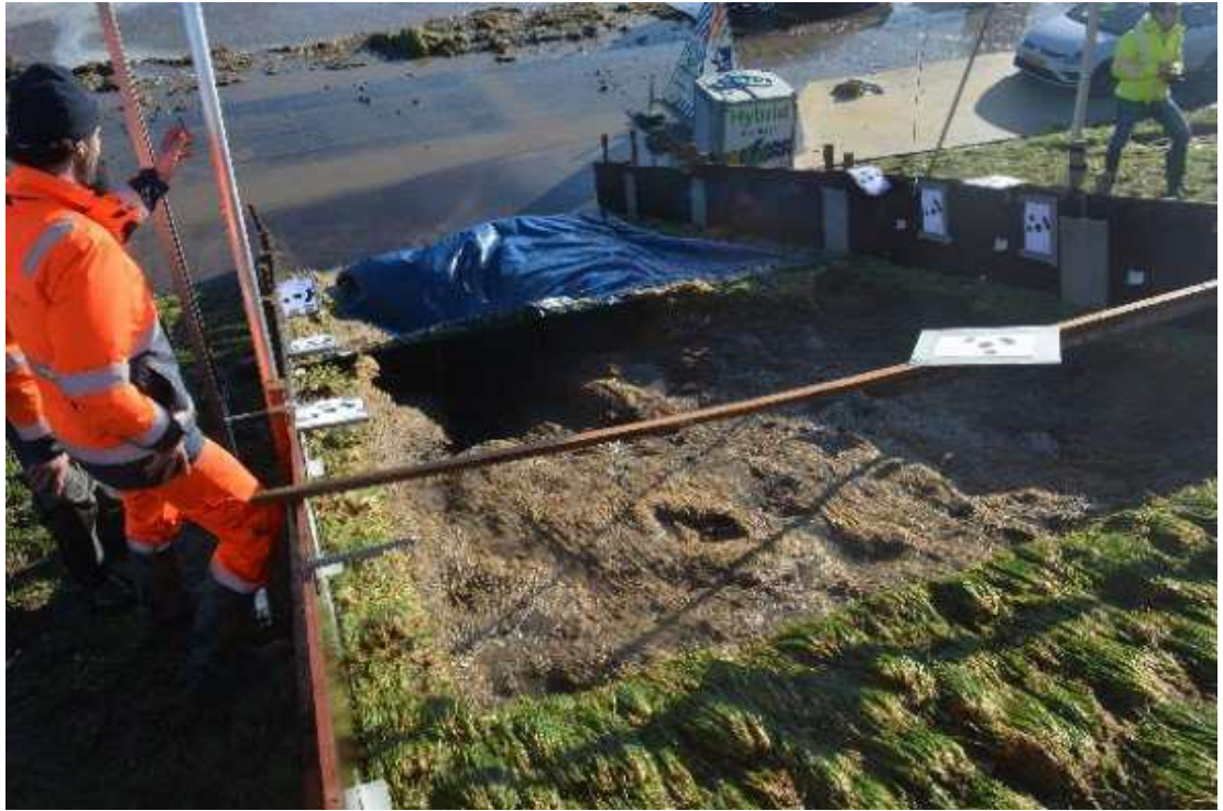
Figure 3.6 Final situation at the end of test 5 (BC2_2).
