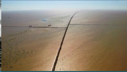
Dept. River & Harbor Engineering
