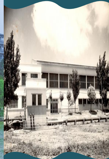
Nanjing Hydraulic Research Institute MWC, MOT
