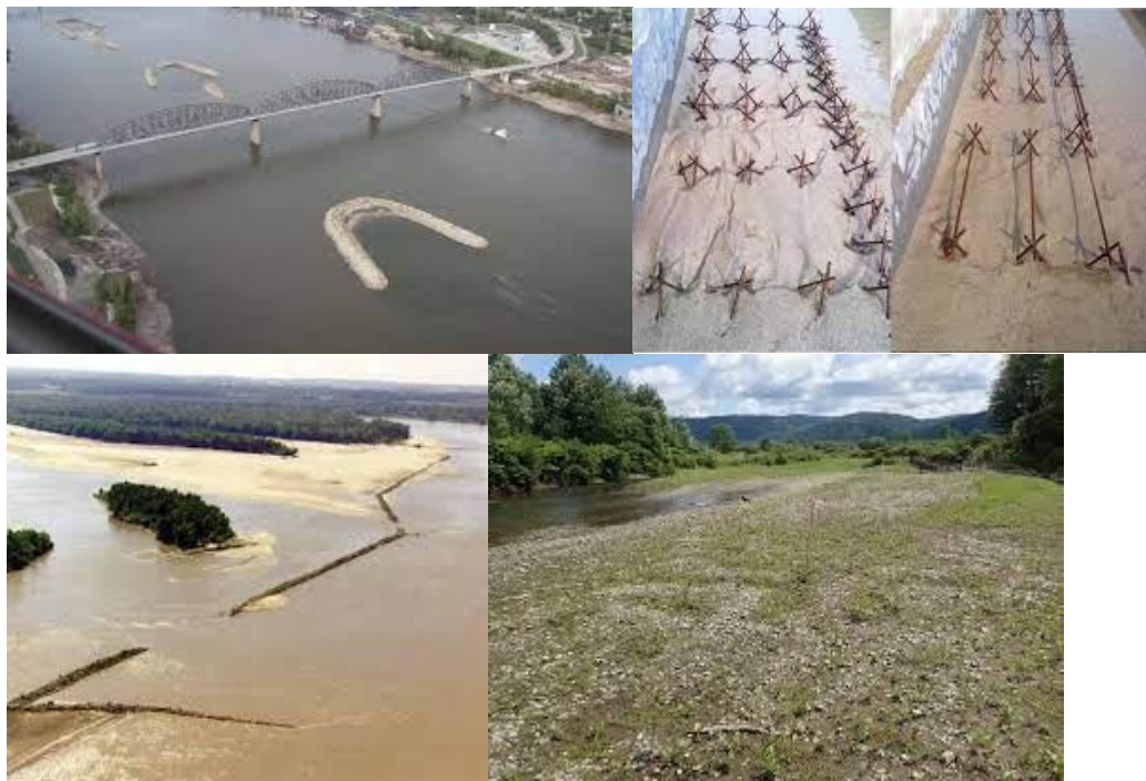
Figure 7-11 Examples of flexible river training structure in order of appearance: Chevron-forming structures ( www.engr.colostate.edu ); tetrahedron frames ( https://link.springer.com/chapter/10.1007/978-981-19-7100-6_17 ); notched closure structure ( www.mvs-usace.army.mil ); gravel bar ( https://guides.nynhp.org/riverside-sandgravel-bar/ )
