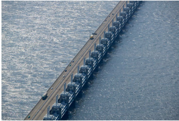
Figure 3.1 Aerial view of the Storm surge barrier in the Eastern Scheldt
