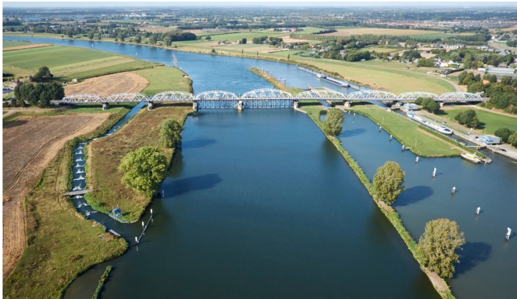
Figure 1.2: [EN] Lock- and weir complex Grave in the river Meuse. [NL] Sluis- en stuwcomplex Grave in de Maas. © Rijkswaterstaat | Joop van Houdt.
