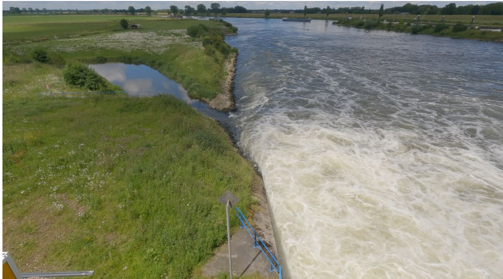
Figure 3.7: [EN] Whitewater near the fishway entrance ( Q \approx 330 \text{ m}^3/\text{s} through the small Poirée weir, June 19 th , 2024). [NL] Turbulente stroming nabij de vistrapingang ( Q \approx 330 \text{ m}^3/\text{s} door de kleine stuw, 19 juni 2024).
