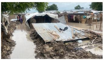
*Figure 2: Kilagaru camp in Dikwa flooded on 06th August 2024. Note the collapsed mud walls and non-durable construction.*
