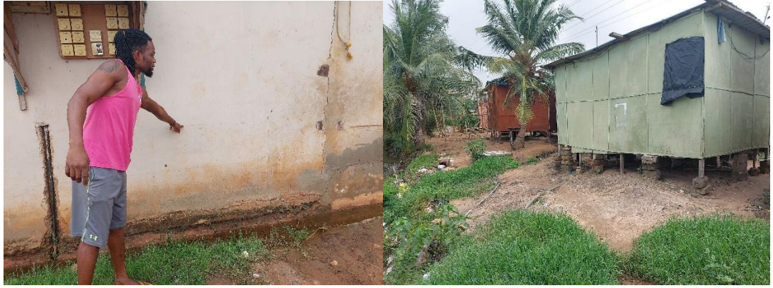
Figure 1. Illustrative housing conditions in flood-prone areas of Accra. Left: residential flood impact, with the reported flood level indicated on the wall. Right: elevated housing as a local adaptation to recurrent flood exposure. The images provide contextual grounding for the proxy-based, distribution-sensitive interpretation of district-level damages.
