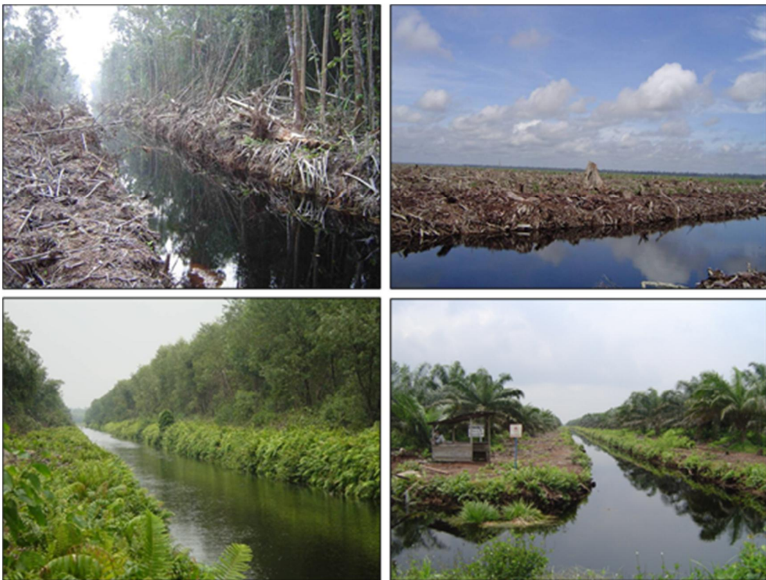
Figure A Canal water depths at 3 to 6 months after canal construction (top left), one to 2 years after canal construction and clearing (top right), in an Acacia plantation more than 6 years after drainage (bottom left) and in an oil palm plantation 18 years after drainage (bottom right). (Photos Hooijer, 2006 -2010).
