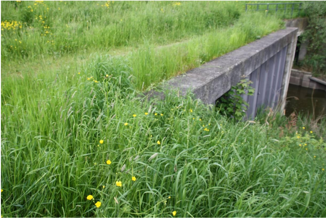
Photo 2.4 Piling sheet at the bottom of strips 1 and 2 (Location 1)
