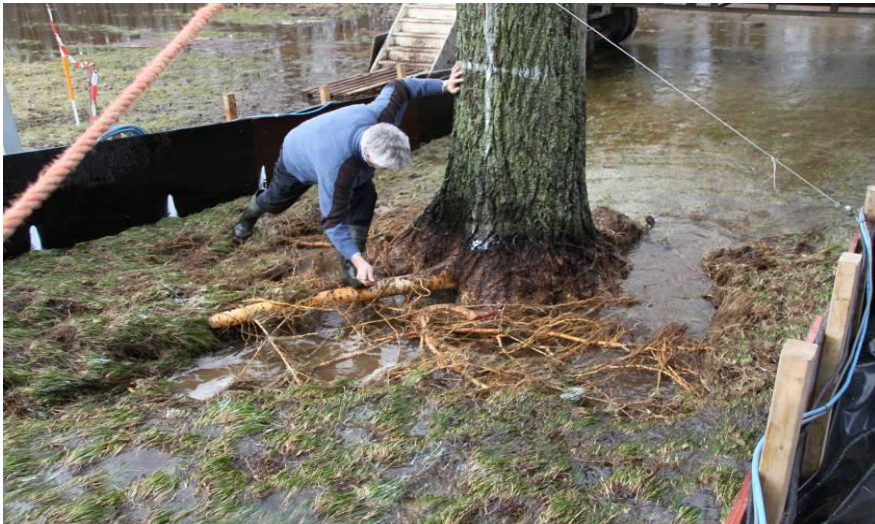
Figure A.3 Erosion at tree; width of test section is 4 m
