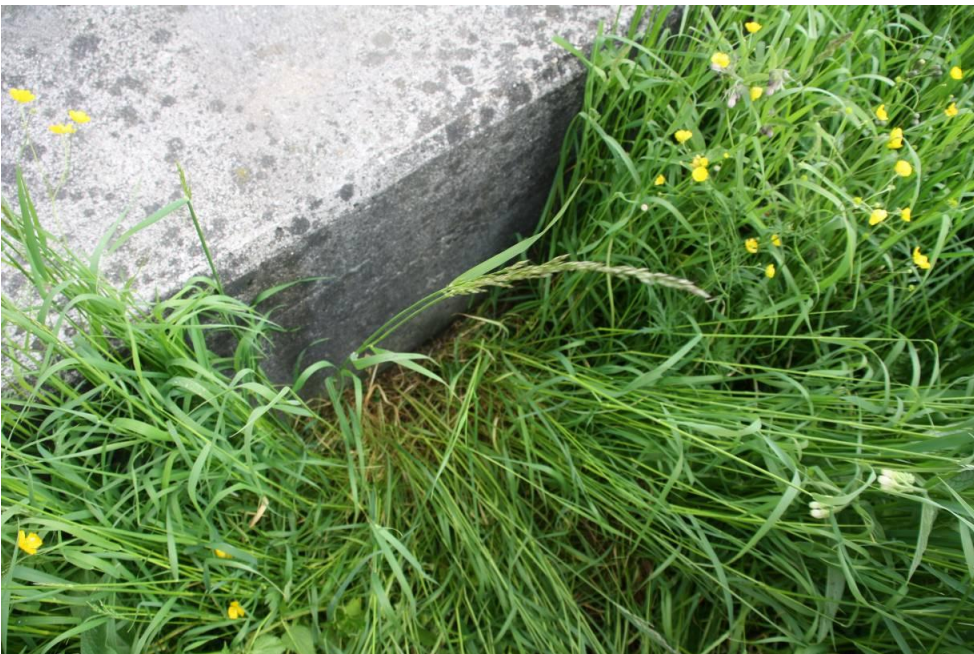
Photo 2.3 Connection of concrete roof of fish ladder to grass cover (Location 1)
