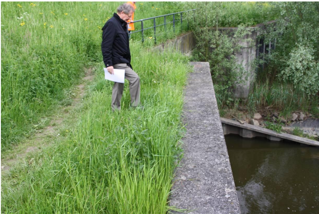
Photo 2.5 Trail between piling sheet and transition of slope to berm (Location 1)
