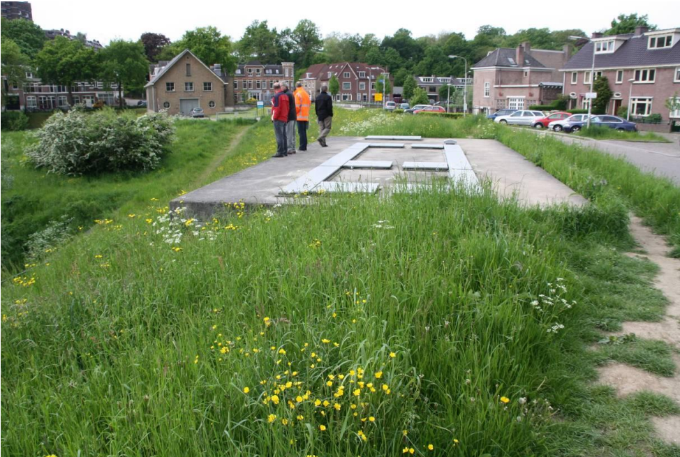
Photo 2.2 Concrete roof of fish ladder (Location 1), Inner side of the dike is on the left
