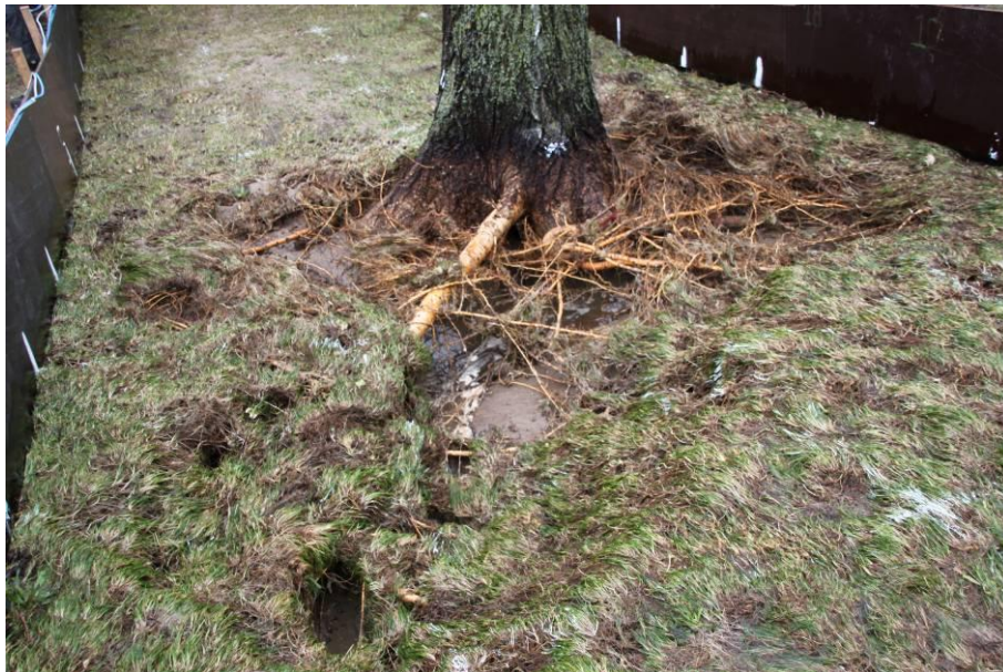
Figure 2.4 Erosion at tree; width of test section is 4 m
