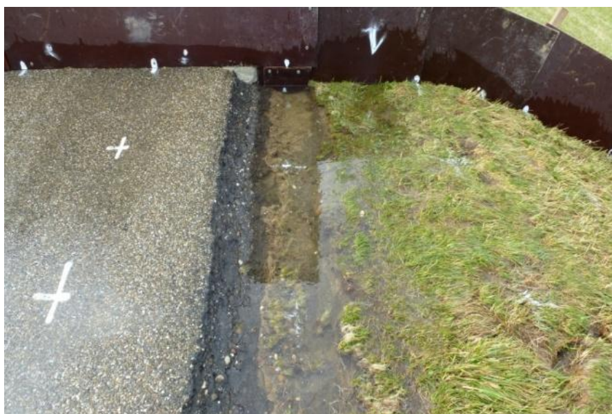
Figure 4.25 Revetment transition from asphalt to grass (Millingen aan de Rijn)
