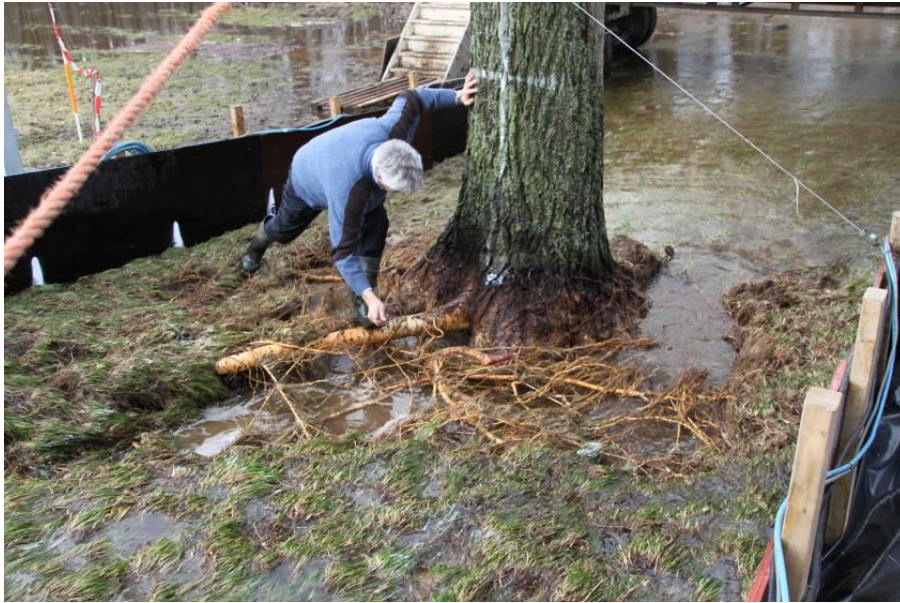
Figure 4.30 Erosion at tree; width of test section is 4 m
