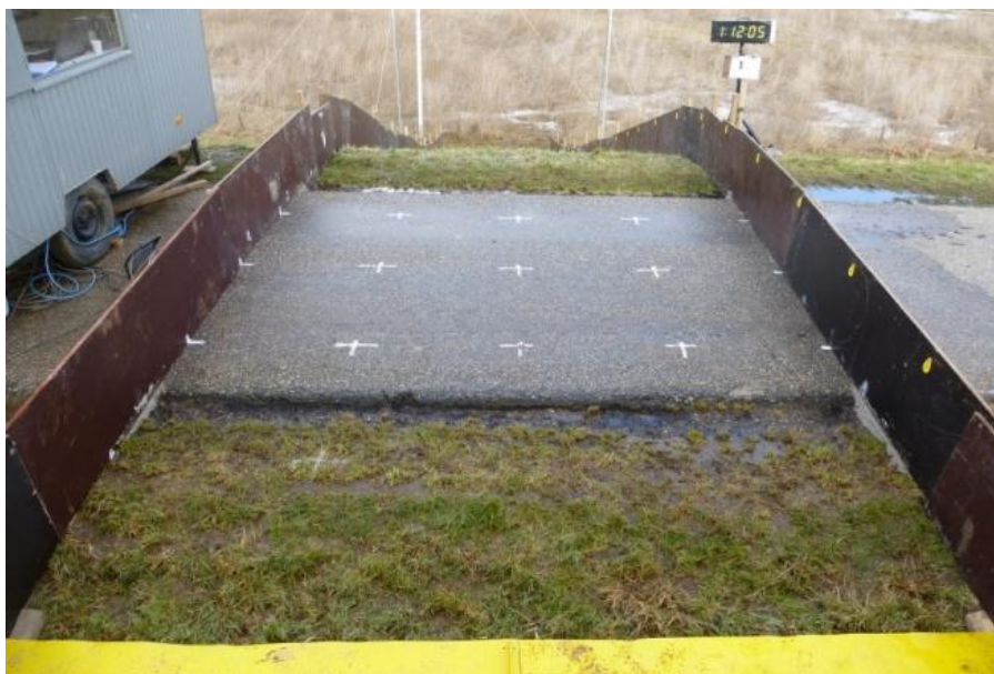
Figure 2.2 Revetment transitions from grass to asphalt and from asphalt to grass
