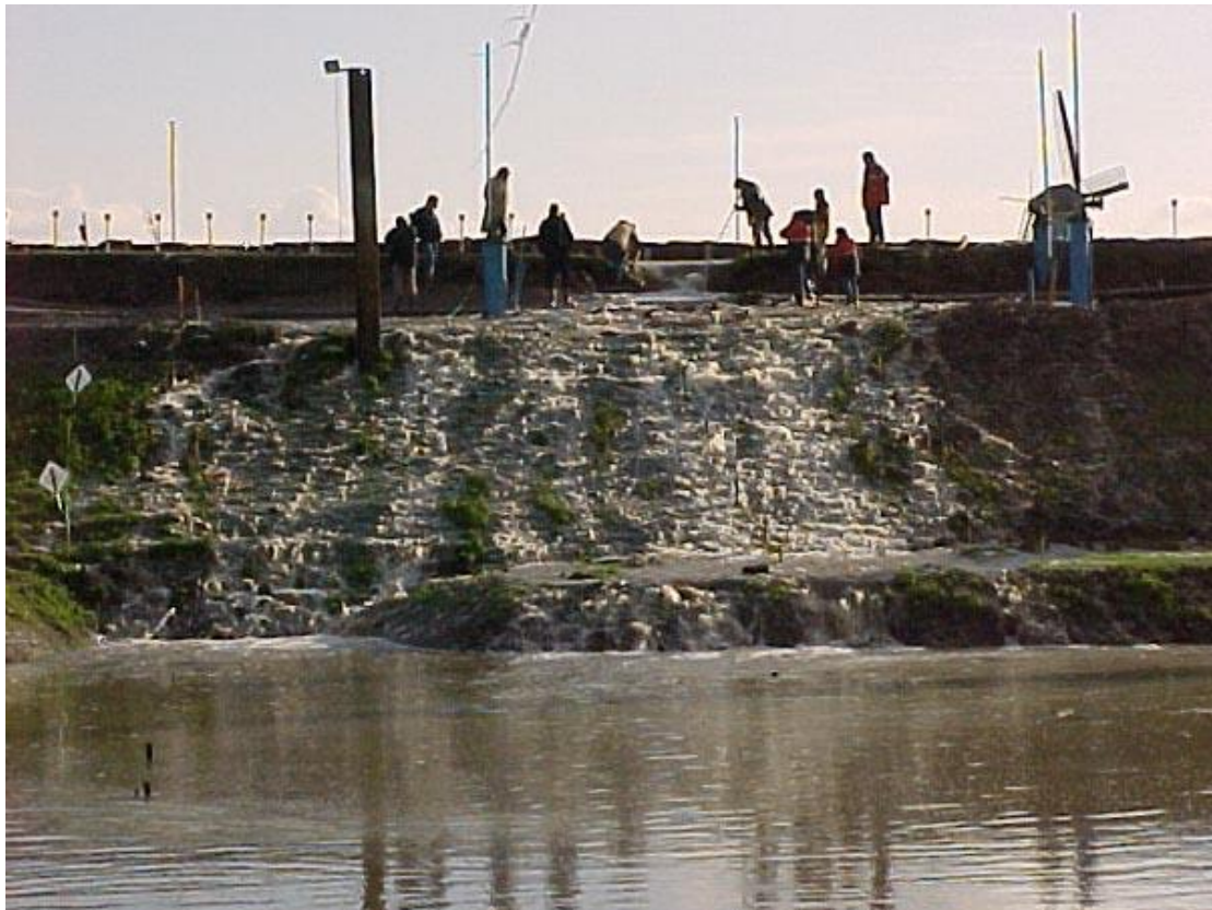
Figure 3.3 Bergambacht overflow test after slip failure test
