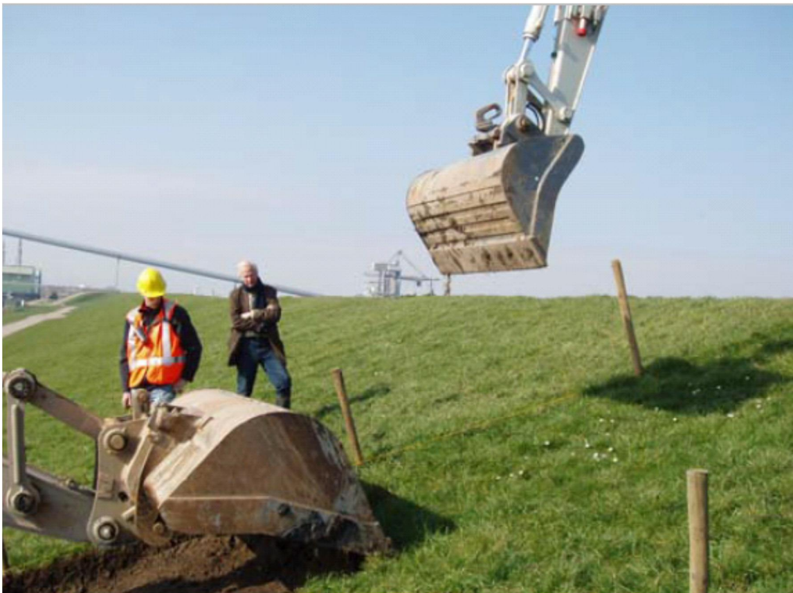
Figure 6.2 Two cranes stripping the sod from the clay (ComCoast)
