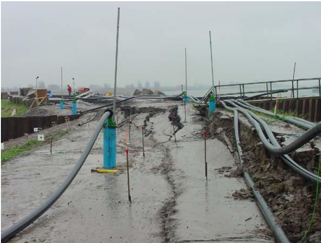
Figure 3.2 Bergambacht slip failure test
