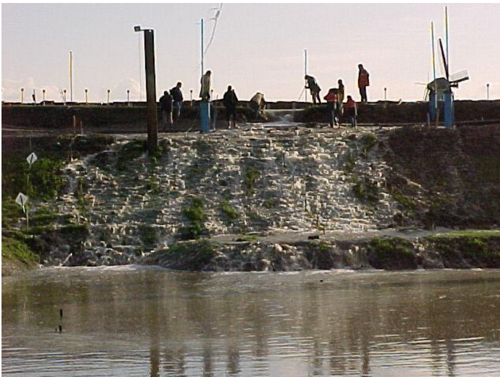
Figure 6.7 Overflow seen from the landward slope
