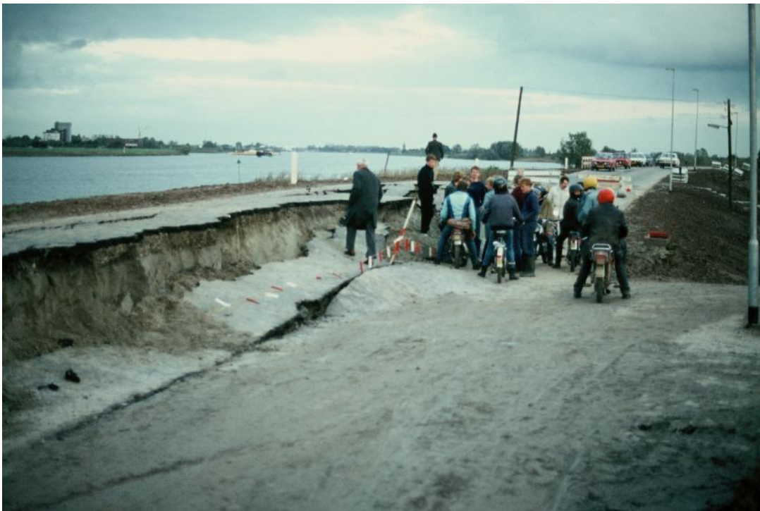
Figure 3.1 Slip failure Sreefkerk
