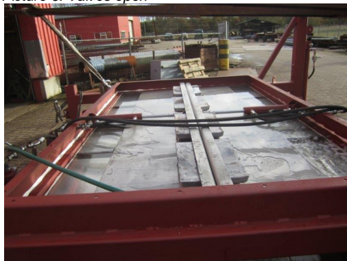
Picture 8. Valves with a few centimetres water
