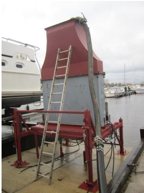
Picture 27. Filling till 3 m water column
