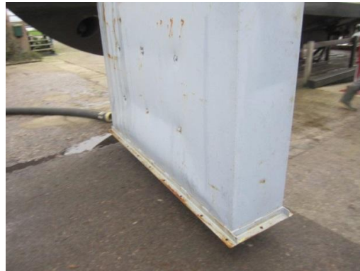
Picture 35. Bended lower module water column
