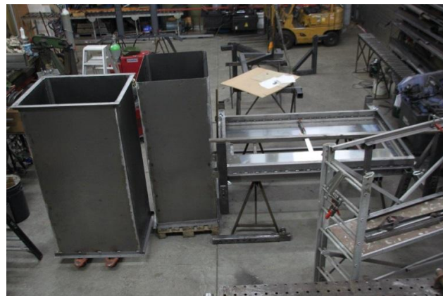
Picture 4. Upper modules and frame for valves
