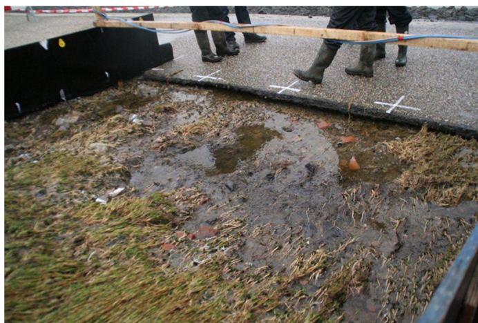
Figure 5.11. Damage to the transition from downward on the seaward slope to the berm. Test on wave overtopping at Tholen
