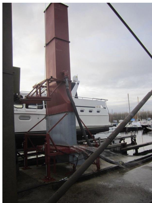
Picture 32. Testing with 7 m water column
