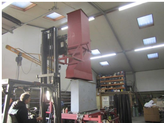
Picture 19. Placing three boxes together
