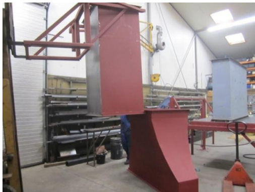
Picture 17. Placing upper box on transition
