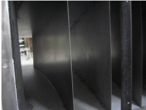
Picture 13 Curved guiding plates at transition
