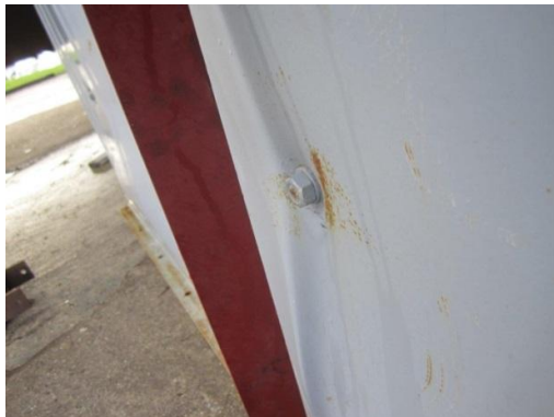
Picture 36. Bended lower module
