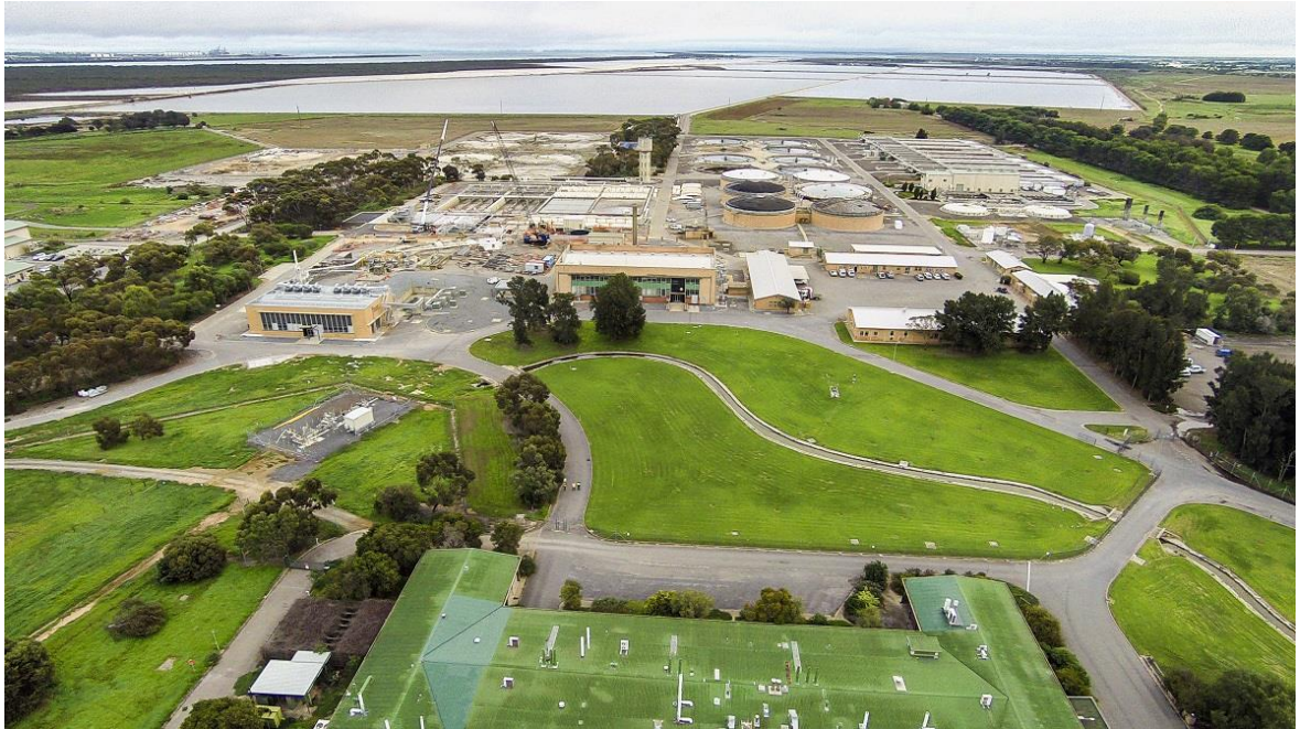
Bolivar Wastewater Treatment Plant – Photograph by SA Water
