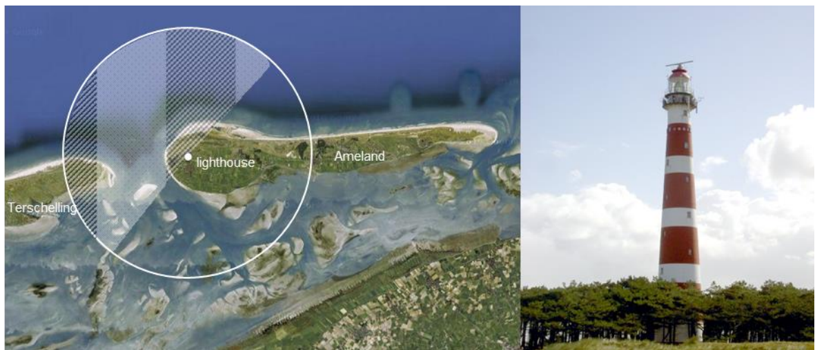
Figure 3.13 Location and approximate range of the lighthouse of Ameland (left) and lighthouse with marine radar mounted on its top (right). From: Swinkels et al. (20??)
