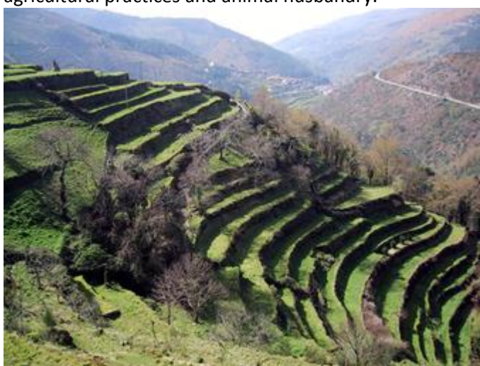
Figure 6.6: The collapsing agricultural terraces of Sistelo (Portugal).
