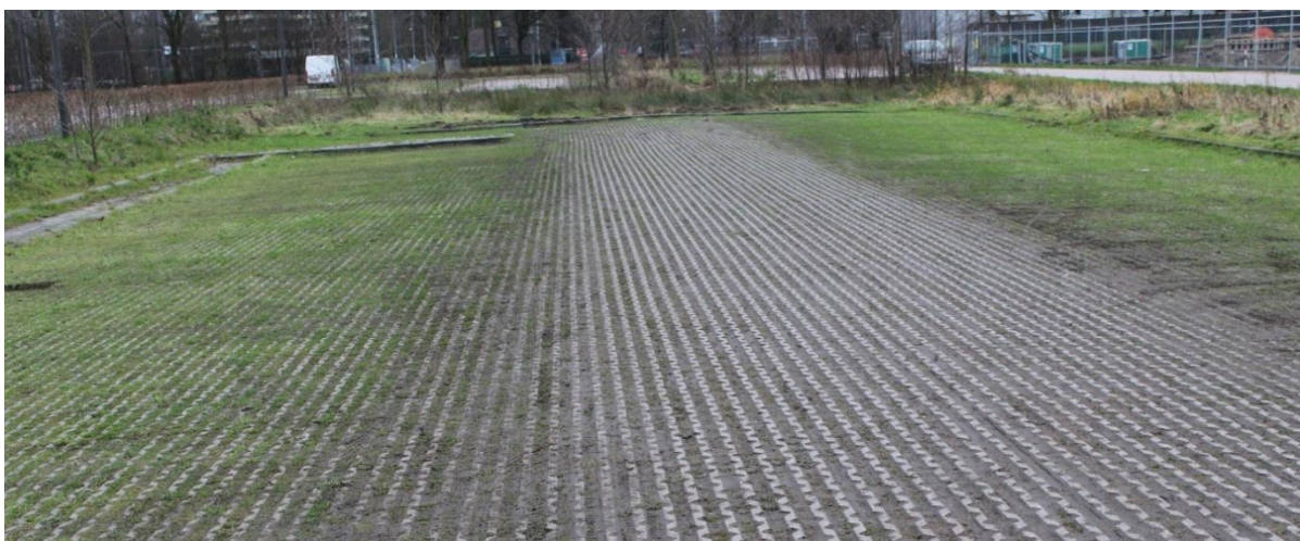
Figure 6.1: Permeable pavement can be applied to reduce the sealing grade of areas that need to be paved due their function (picture from EEA, 2016a).
