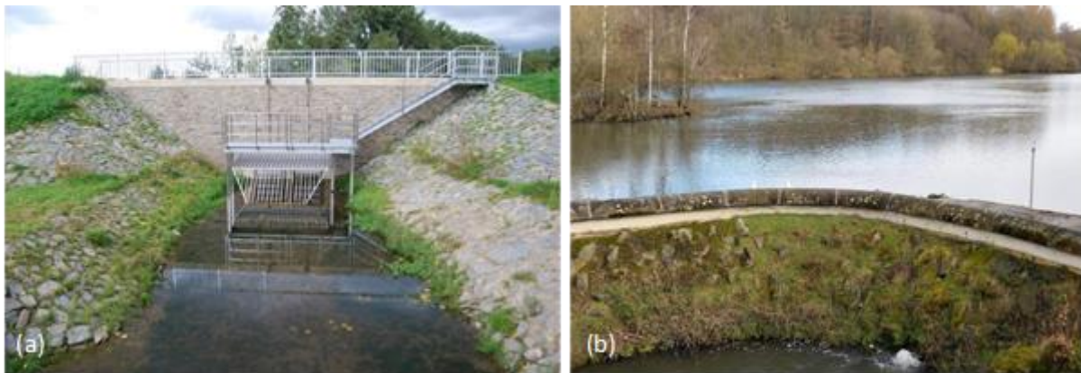
Figure 2: Flood control reservoirs, (a) flood retention basin Düren, (b) flood retention basin Broicherbach
