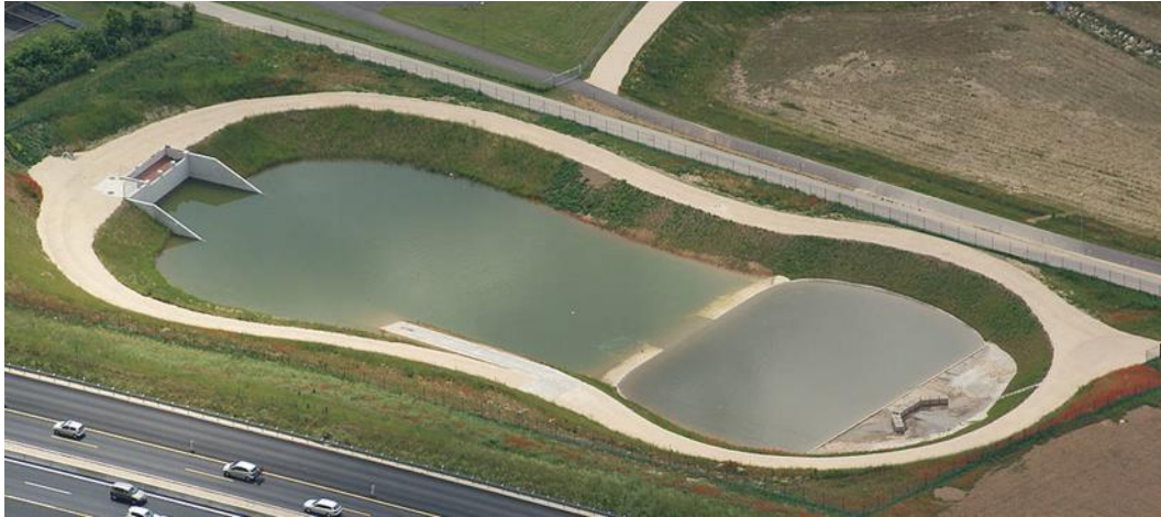
Figure 3: Rainwater retention basin Ulm
