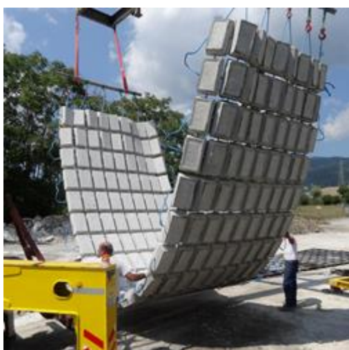
Figure 11.4 Cable-connected block mattress (courtesy of Maccaferri).
