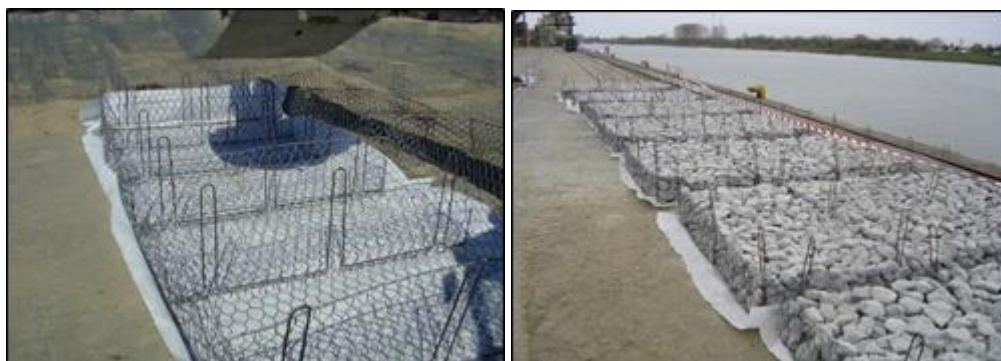
Figure 11.26 \Omega -shaped lifting re-bars for gabions and gabion mattresses.
