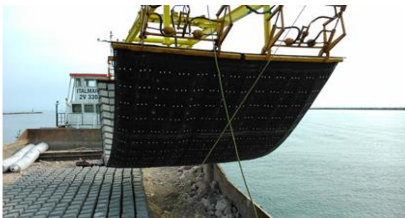
Figure 11.5 Geotextile-bonded block mattress (courtesy of Maccaferri).
