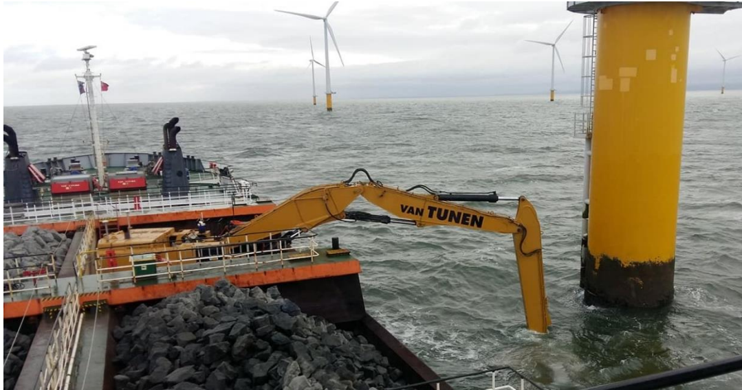
Figure 7.7 Crane Vessel (courtesy of Van Oord)
