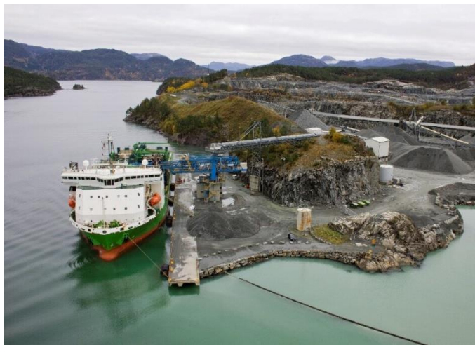
Figure 7.5 Typical loading site (courtesy of DEME offshore).
