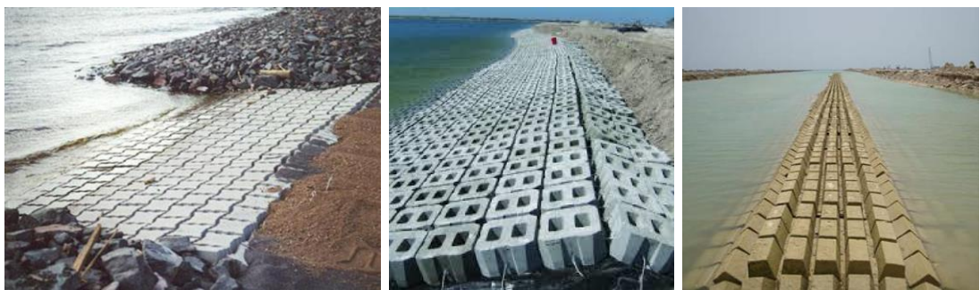
Figure 11.1 Examples of block mattress functions: boat landing (left, www.conteches.com ), embankment protection (middle, www.acfenvironmental.com ) or pipeline protection (right, www.geosynthetica.net ).
