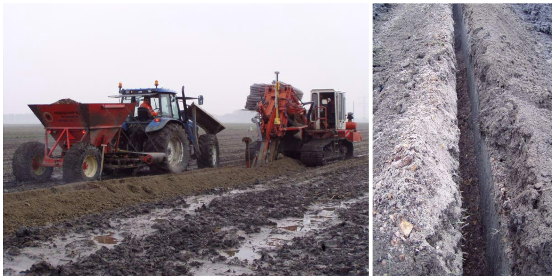
Figure 1. Construction of drain enveloped with wood chips.
