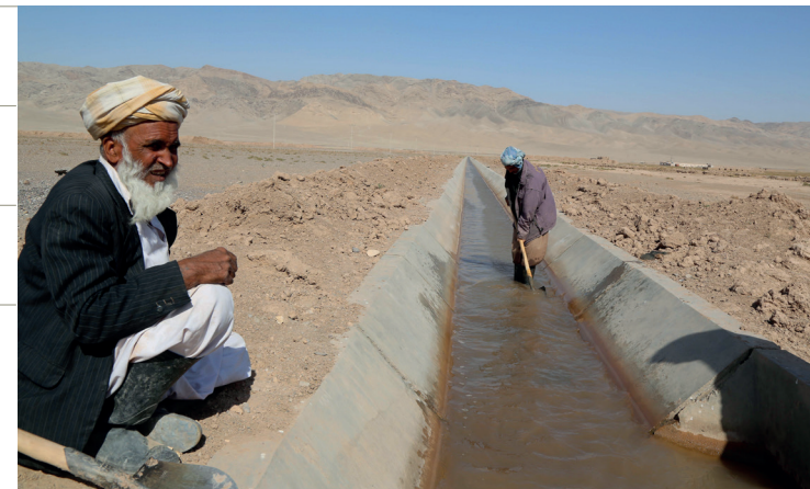
◀ Cemented irrigation channel
