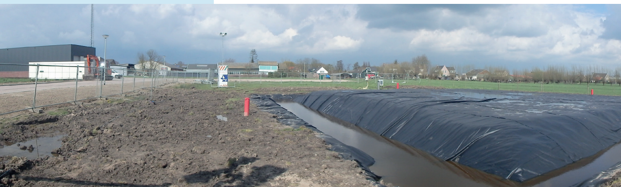
Vacuum trial at Bleskengraaf
