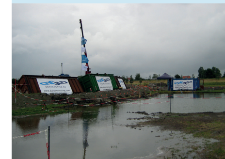
Failure during full-scale testing of dike with JLD Dike Stabiliser (hidden in the ground)
