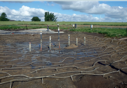
Vacuum trial at Schardam using the new Beaudrain S technique
