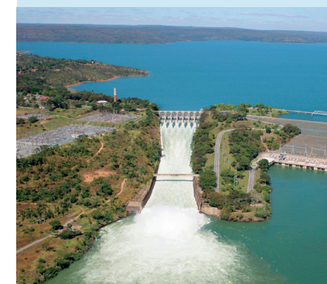
Hydropower optimisation for the Três Marias dam in Brazil (source: Universo Cemig, Dec. 2015)
