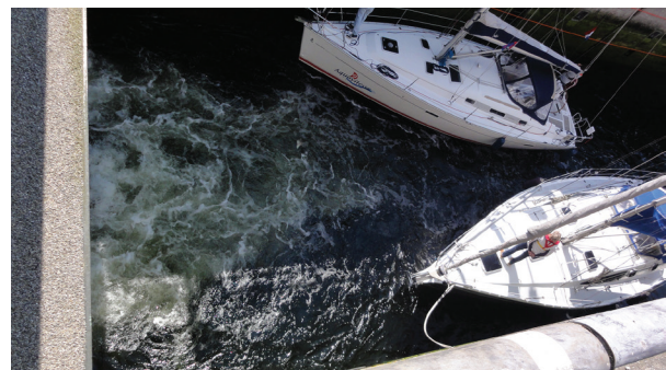
The filling discharge at the water surface for the Krammer recreational lock, Netherlands
