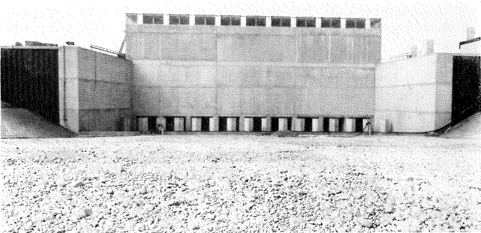
Photo 7. The sluiceway viewed from the storage basin.
