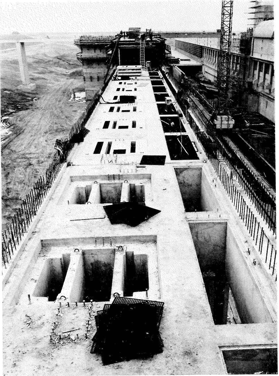
Photo 11. The lock wall illustrating the recessed engine house. The valve slots are clearly visible on the floor.
