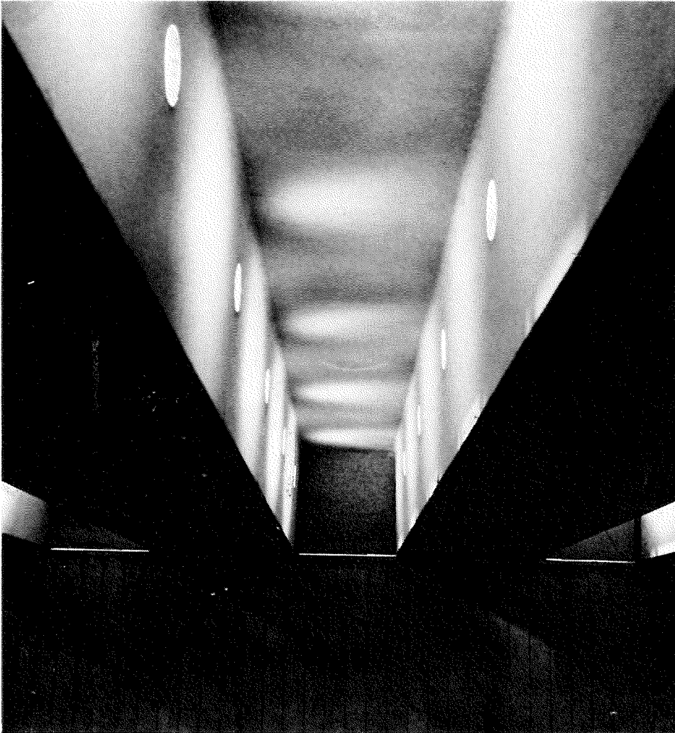
Photo 3. Detail of floor beam.
