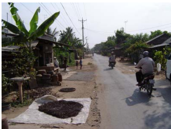
c. Paved road in zone A
