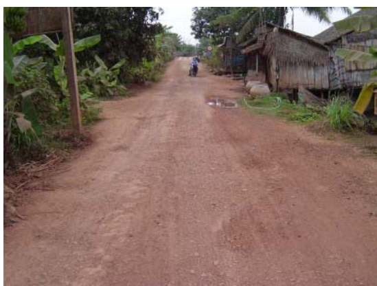
a. Unpaved road in zone C
