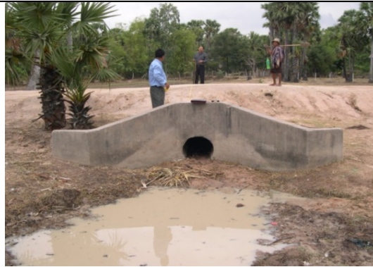
Figure 5: Example of a small culvert
