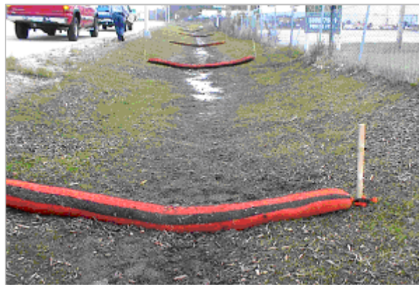
Figure 3.4 Installation of filter socks in a road ditch, Indiana, United States
