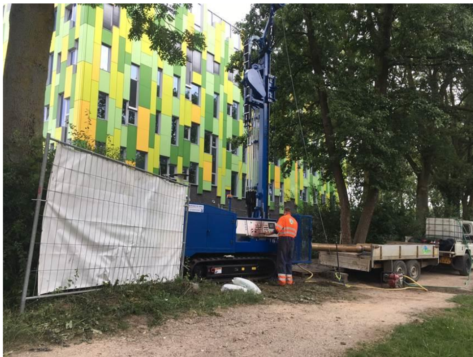
Figure 4: Installation of the monitoring well
