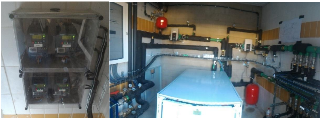
Figure 8. Impression of plant room
