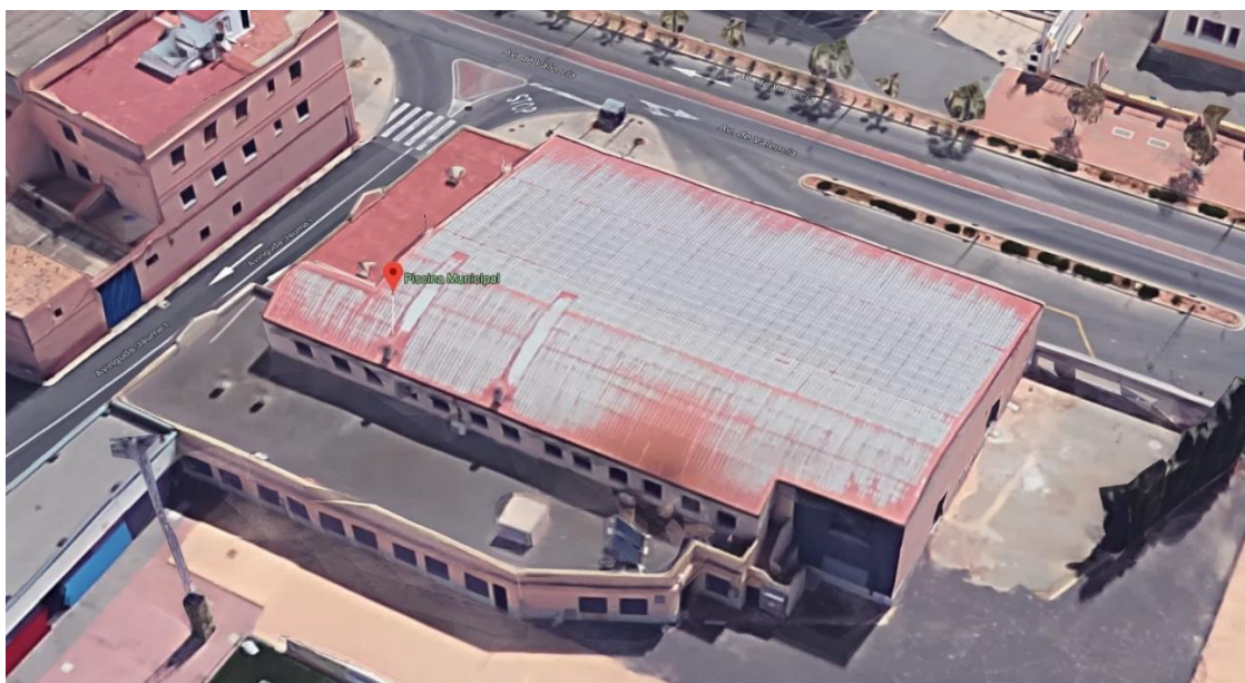
Figure 3. aerial view of the swimming pool
