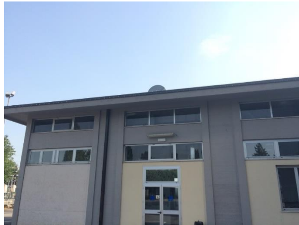
Figure 2. Entrance of the changing rooms building.
