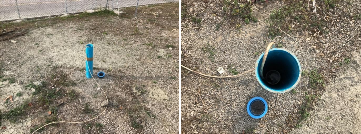
Figure 22. One of the monitoring wells during a constant flowrate pumping test.
