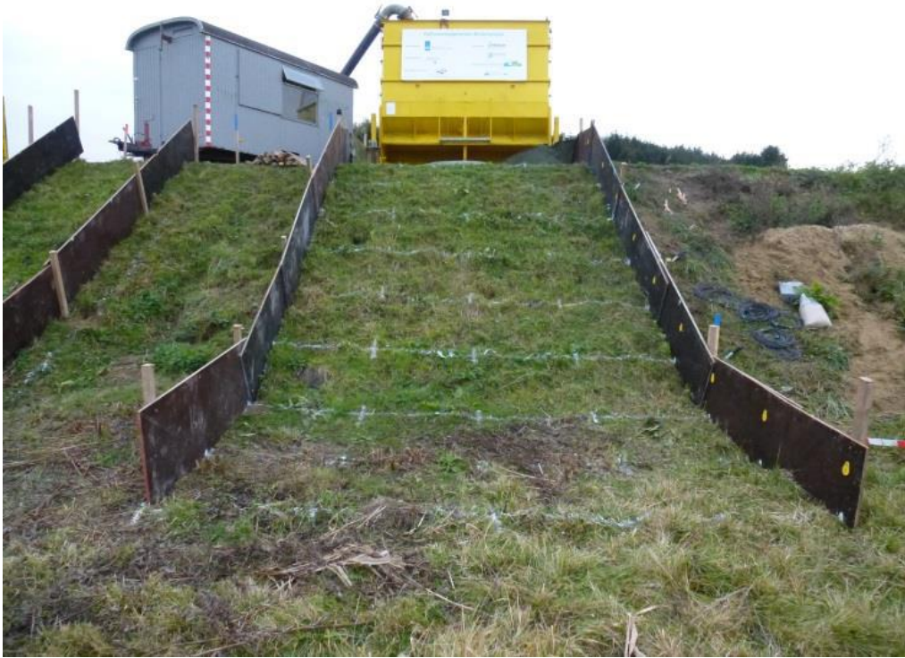
Figuur 70 Nulsituatie grasbekleding Teststrook I (Infram, 2015, Factual report)
