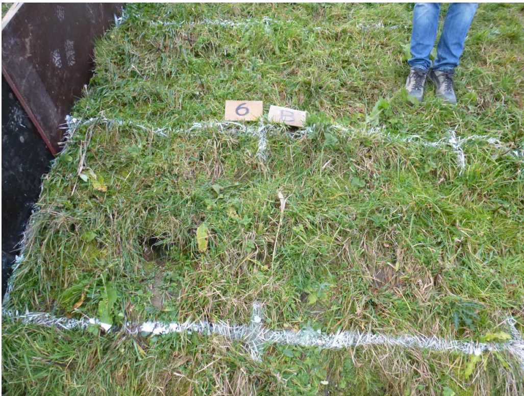
Figuur 71 Nulsituatie grasbekleding Teststrook I vak 6B (Infram, 2015, Factual report)
