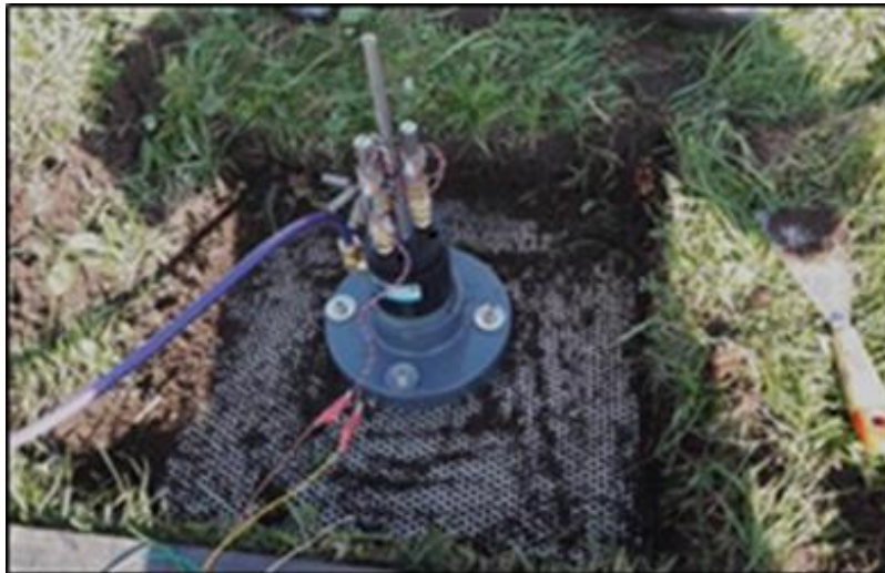
Figure 6 Image of buried perforated stainless-steel plate/mesh to which the head assembly of the extensometer is attached (location Rouveen, NOBV).
