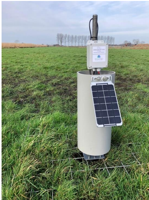
Figure 7. 2-point extensometer at Zegveld which uses a magnetostrictive linear position sensor to monitor the deformation (Gé van den Eertwegh, KnowH2O).
