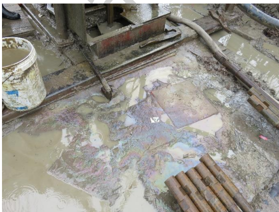
Figure 11: Example of bad practice with the drilling site contaminated by hydrocarbons (Source: BGR, 2020)
