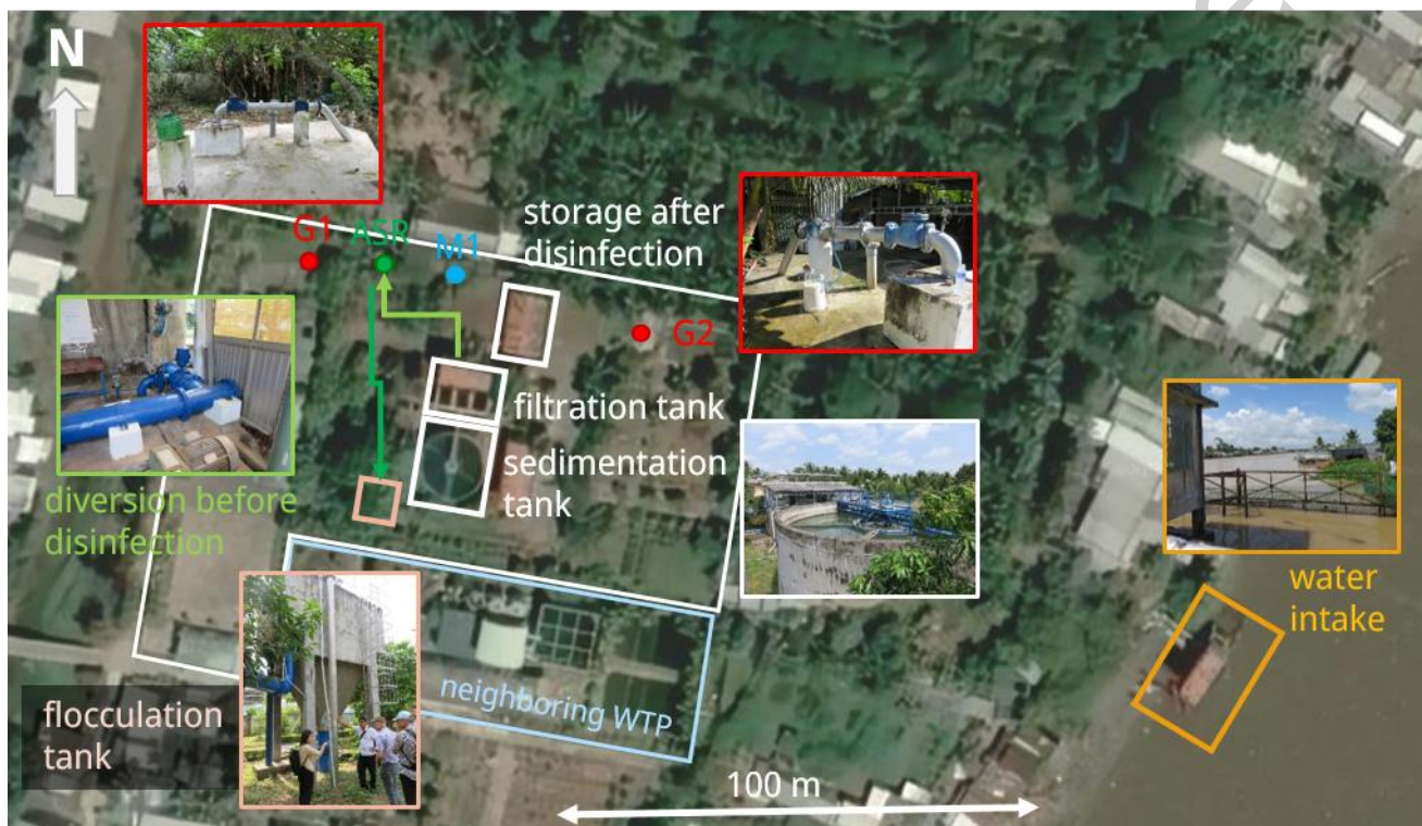
Figure 3: Overview of water treatment plant (WTP) of HAWASUCO in Nga Bay City (white outline) showing the location of existing infrastructure and the neighbouring water treatment plant (light blue outline) in cooperation with HAWASUCO. G1, G2: existing production wells, M1: monitoring well drilled in January 2024 by the project, ASR: proposed location for drilling ASR well. Source: GoogleEarth, Photos BGR.
